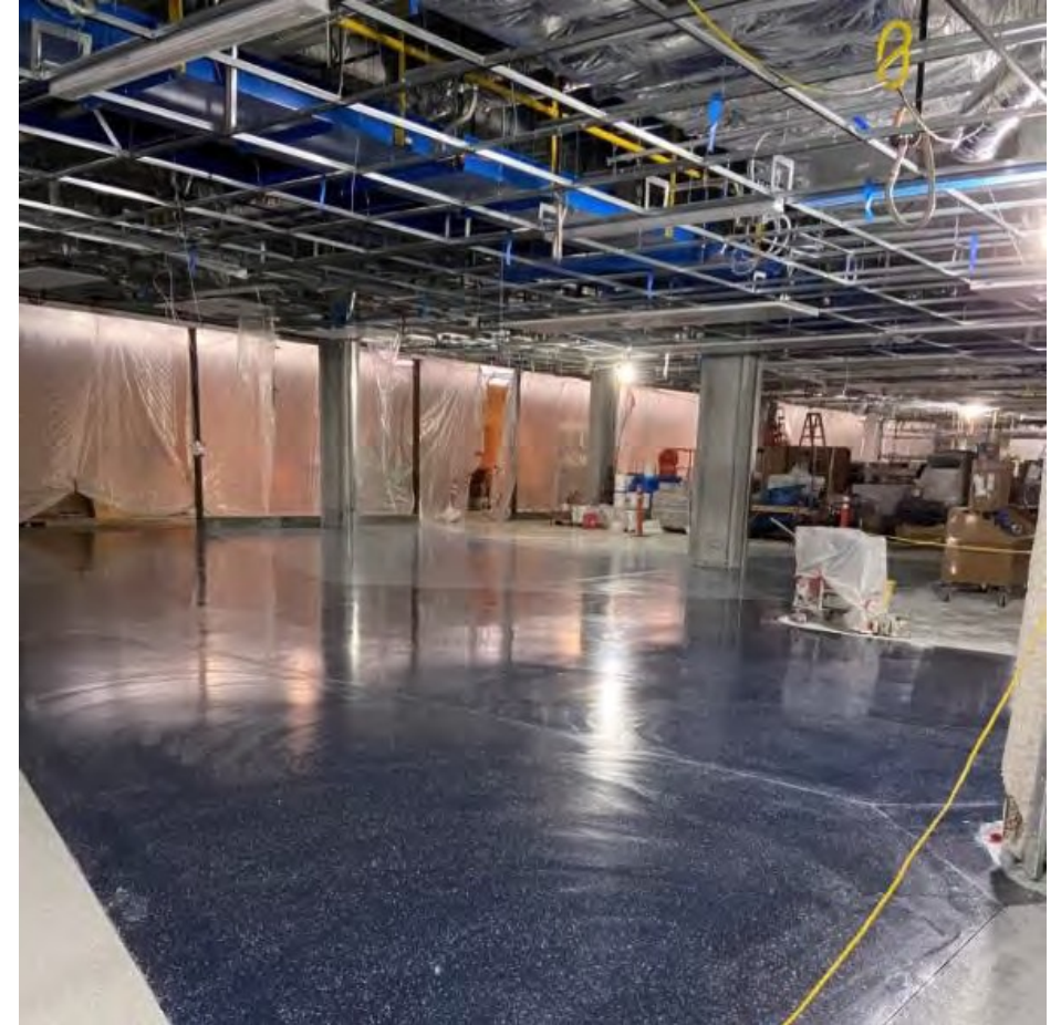
Interior Level 2 – Overhead work, ceiling grids and terrazzo polish
