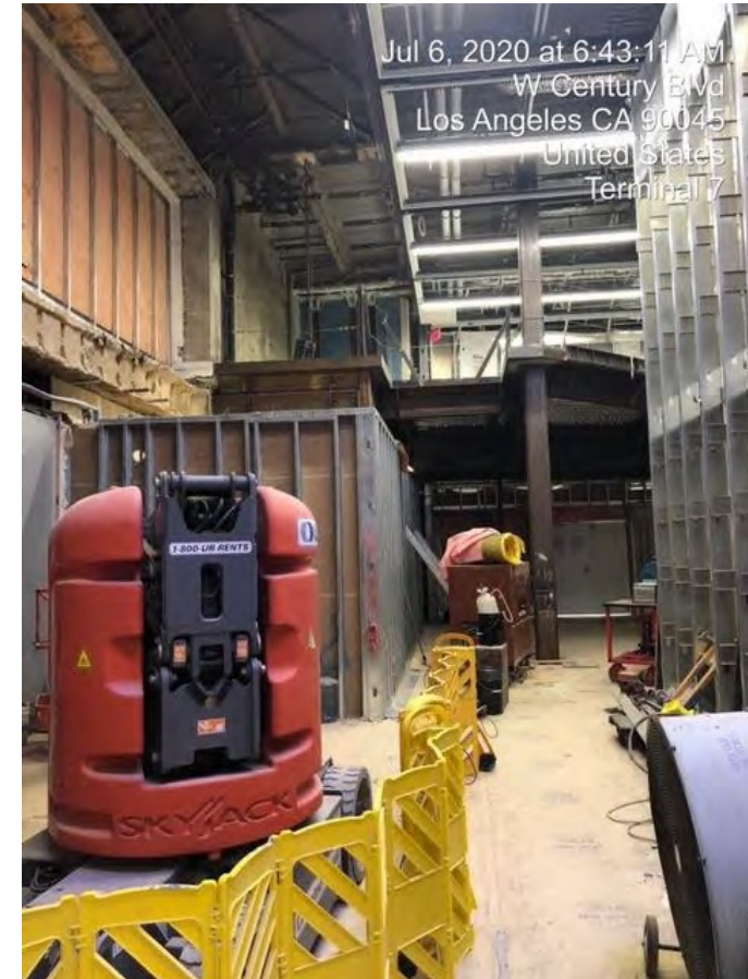
Steel erection for Vertical Transportation
