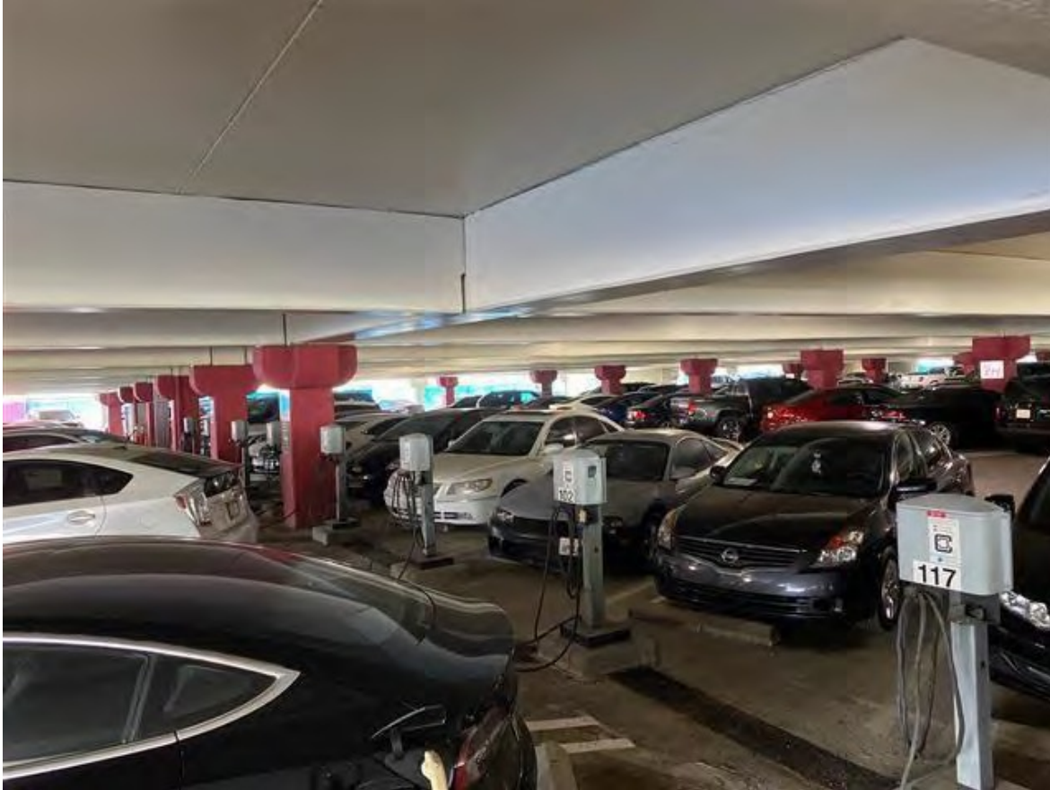
New EV Chargers within Parking Structure 1
