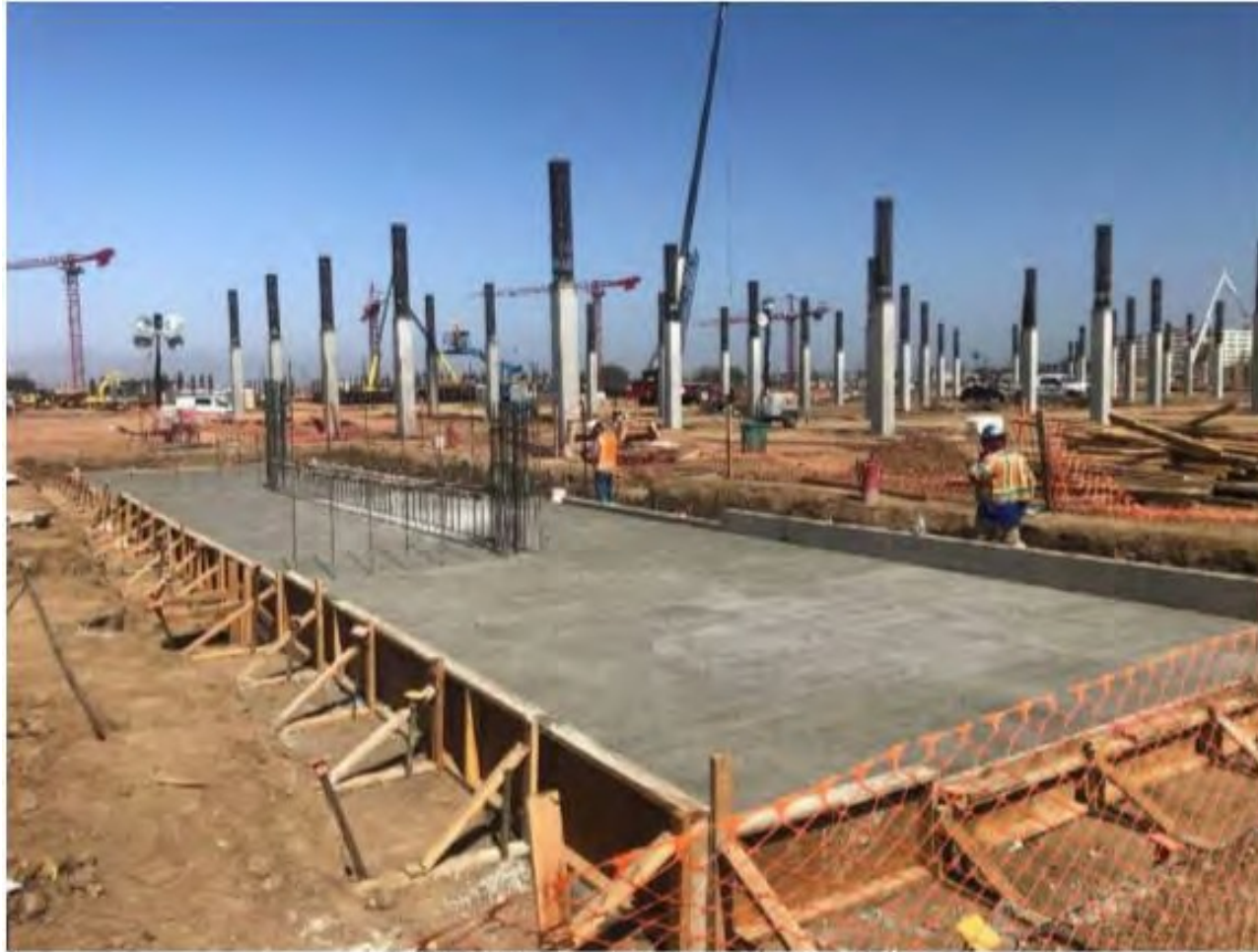
A: QTA – Foundation and shear wall at Stairwell #8
