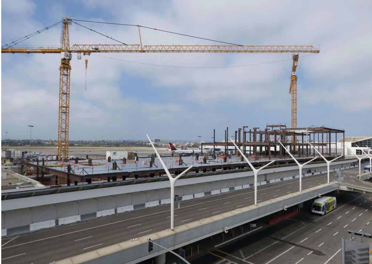
Looking North from CTA – Erection of Structural steel
