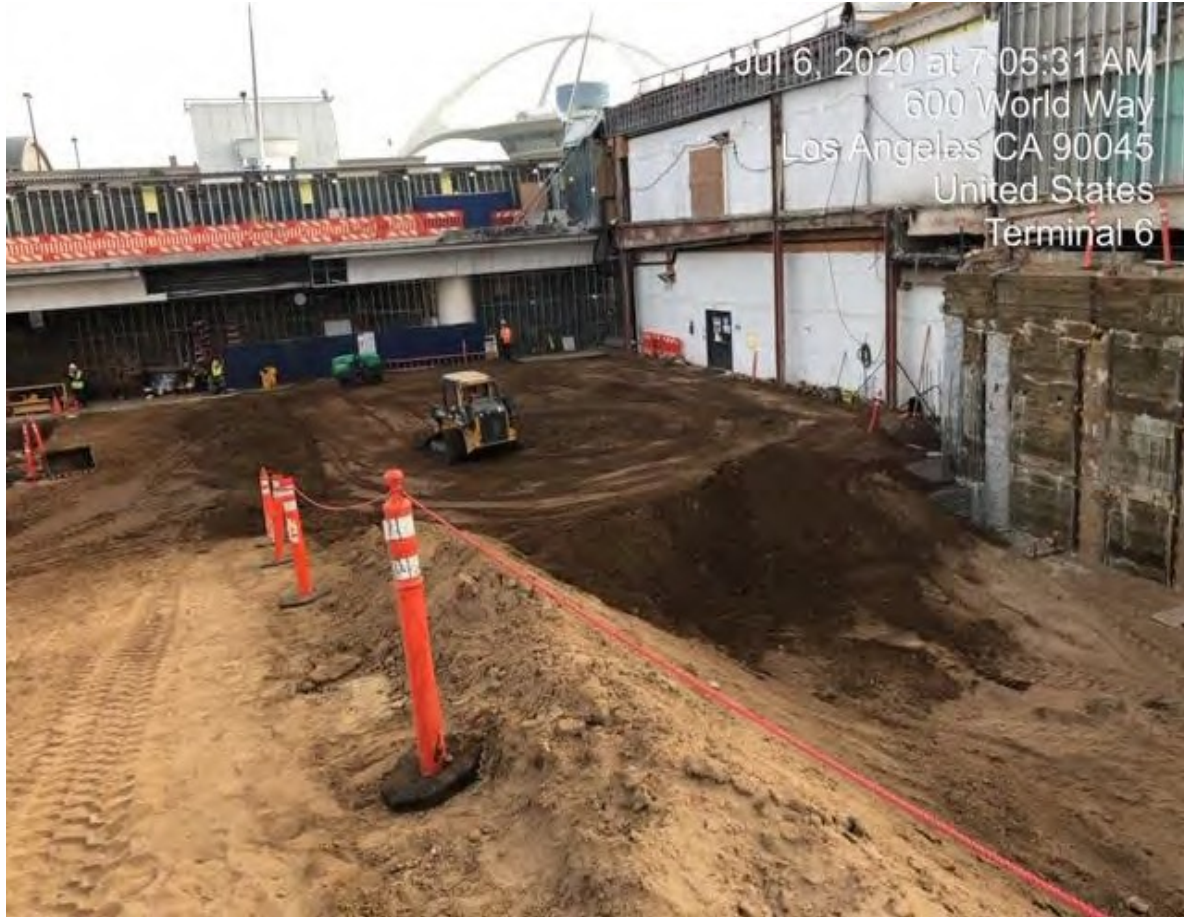
Building pad in preparation for foundation excavation
