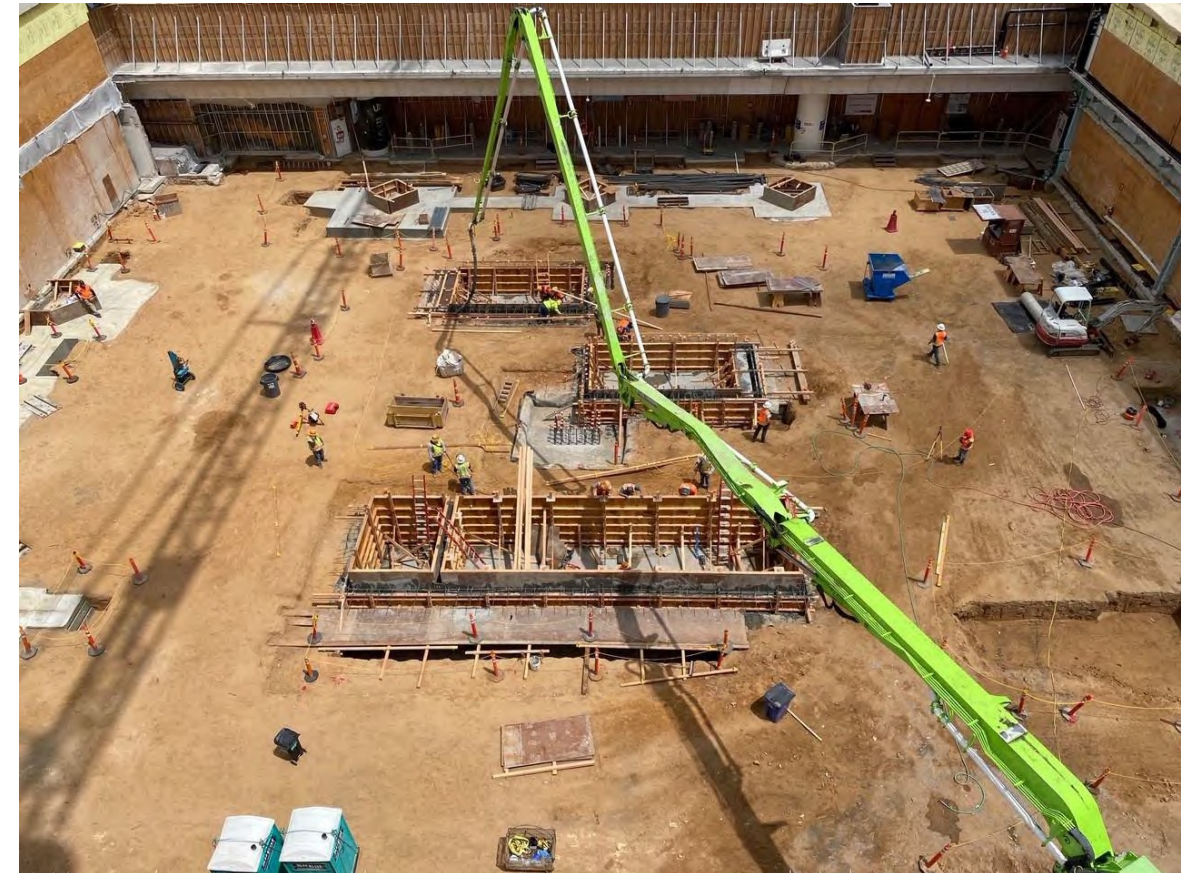
Looking North from Airside – Foundation work for Elevator/Escalator pit
