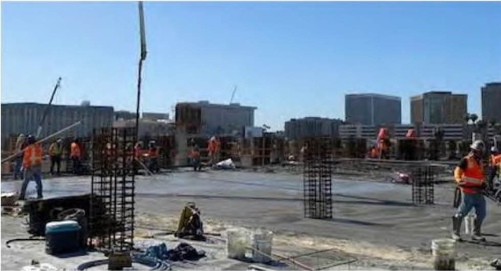
Building C – Looking South East – 2 nd level concrete placement
