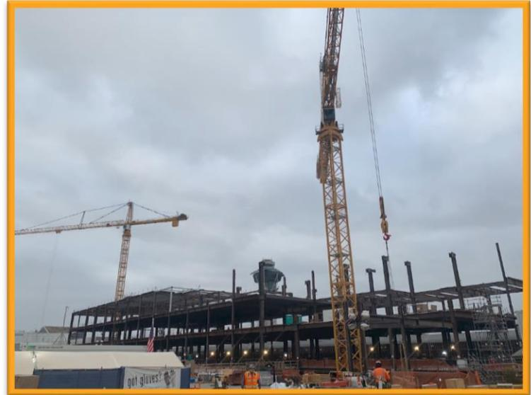
*Right: Future Terminal 2 / 3 Head House during foundation work and steel erection
