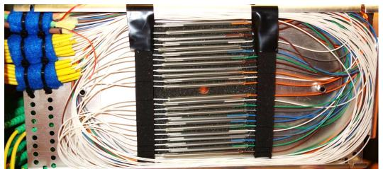
Typical fiber splice tray with fusion splices.
