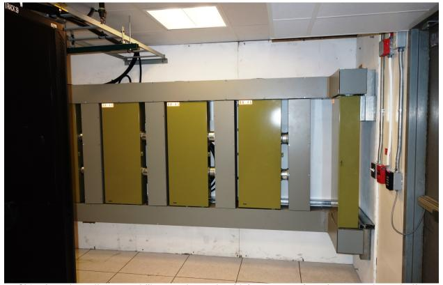
Side view of a wall-mounted fiber patch panels with interconnecting wireway and stand-offs.
