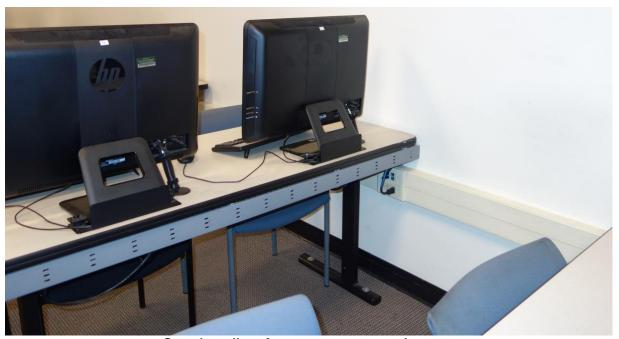
Sample wall-surface-mount raceway shown.
