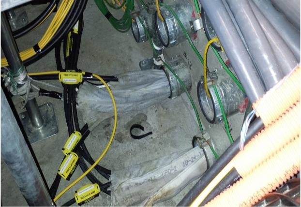
A minimum of one conduit shall have (3) 3", 3-cell, Maxcell fabric innerducts per ductbank run.
