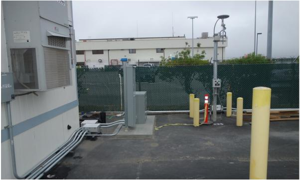
A sample of a temporary conduit installation using galvanized rigid conduit.
