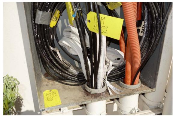
MaxSpace Recovery process: Three innerducts have been removed and two Maxcell's installed.
