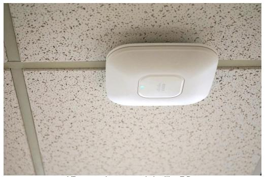
A/P mounted on suspended ceiling T-Bar.
