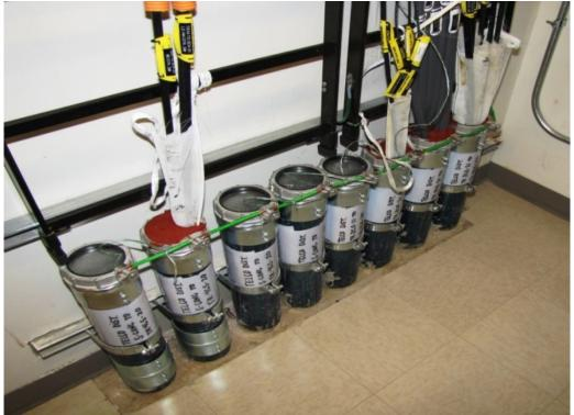
Conduit stub-ups shown secured to wall-mounted strut.
