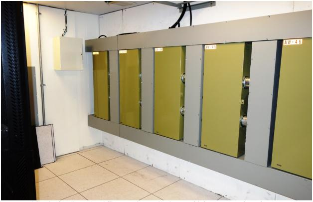
A bank of wall-mounted fiber patch panels shown with interconnecting wireway.
