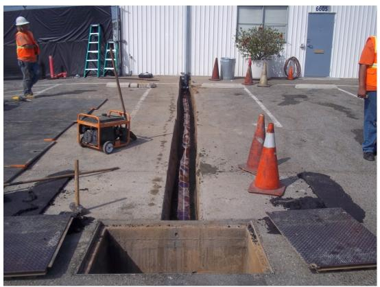
Underground detectable identification tape installed.
