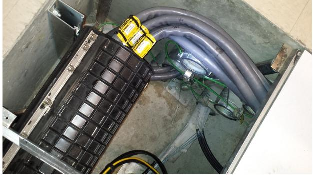
A splice case shown in a conduit well.
