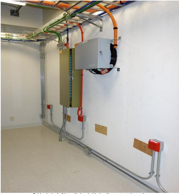
Cable slack shall be coiled up behind wall-mount patch panels.
