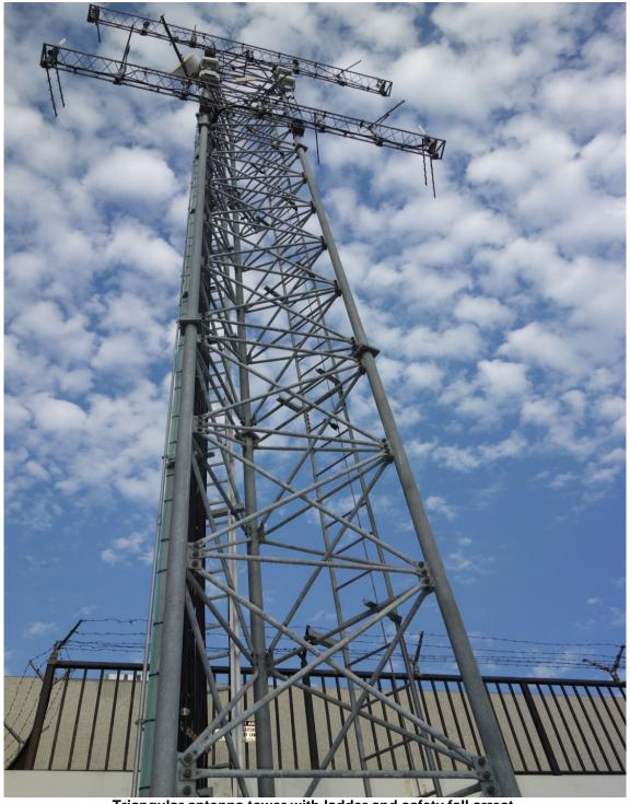
Triangular antenna tower with ladder and safety fall arrest.
