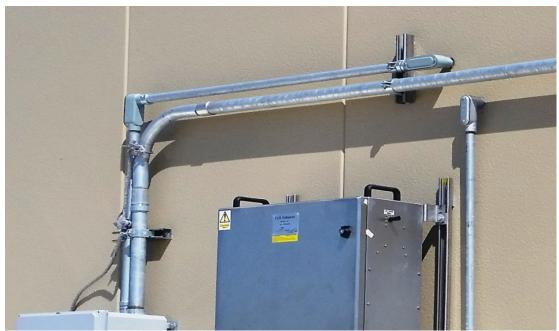
Conduit bodies/condulets used for copper cables.
