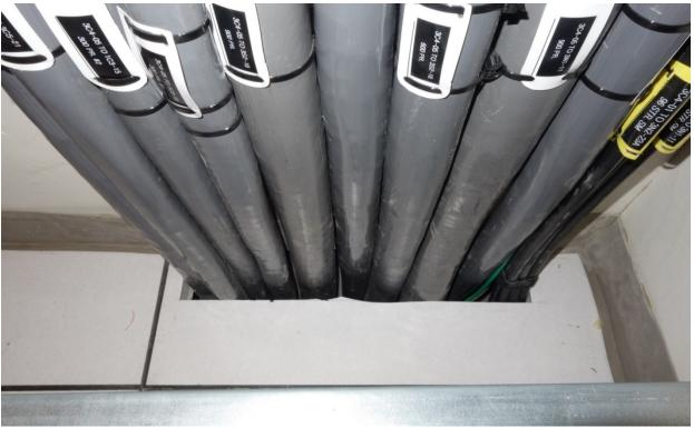
Backbone inside plant CAT 3 copper cables being distributed from an MPOE to local IT Rooms.
