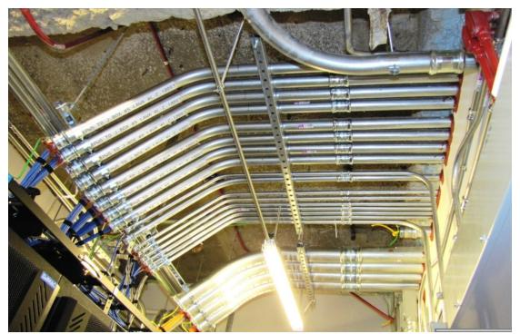
A neat professionally-installed and labeled horizontal conduit bank with bushings is shown.
