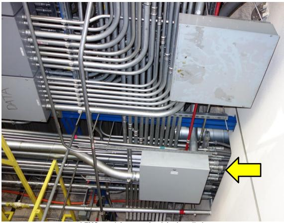
LFMC conduit expansion joint installed.
