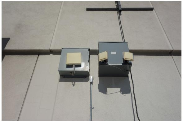
Multiple A/P's are shown mounted on an exterior wall.
