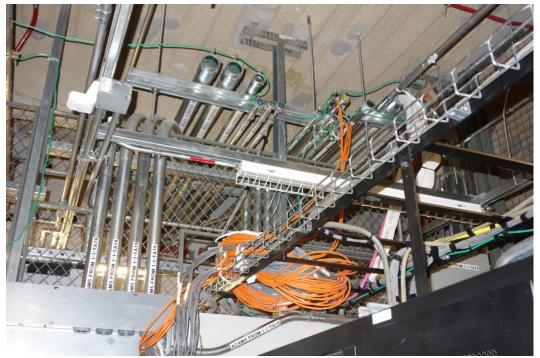
Wire Basket shall be attached to Cable Tray or Ladder Rack. Cable waterfalls are required.
