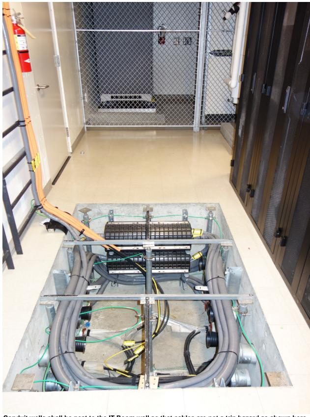
Conduit wells shall be nest to the IT Room wall so that cables are not a trip hazard as shown here.
