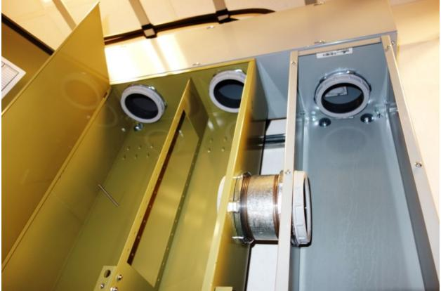
Conduit chase nipples shown connecting patch panel to top and right wireway.
