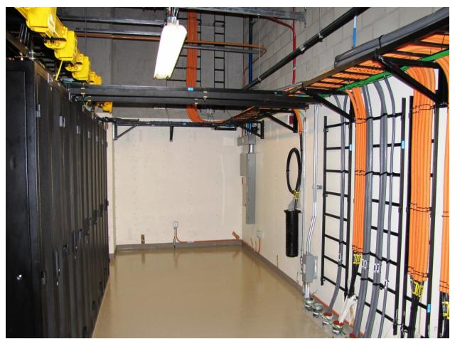
In IT Rooms, vertical Ladder Rack is required to secure cables that transition to floor conduits.
