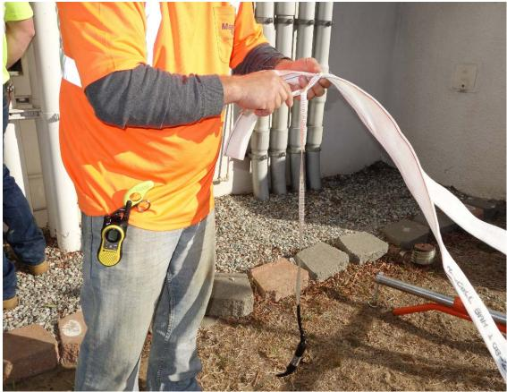
MaxSpace Recovery process: The fabric innerduct is being prepared to replace the HDPE.
