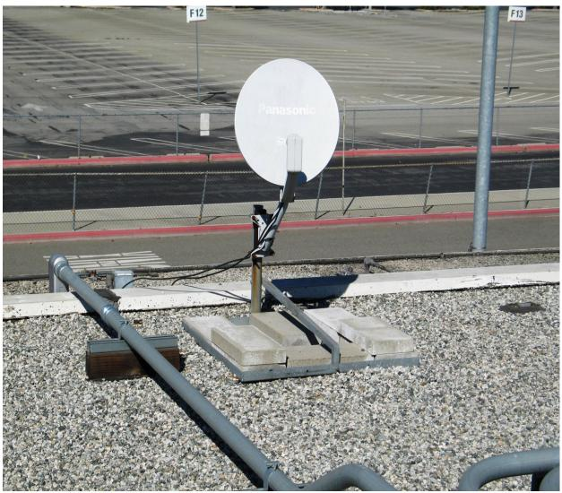
A sample small non-penetrating rectangular-base surface roof mount is shown.
