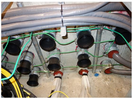
Conduit well showing cable support, fabric innerduct, firestop, and conduit plugs.
