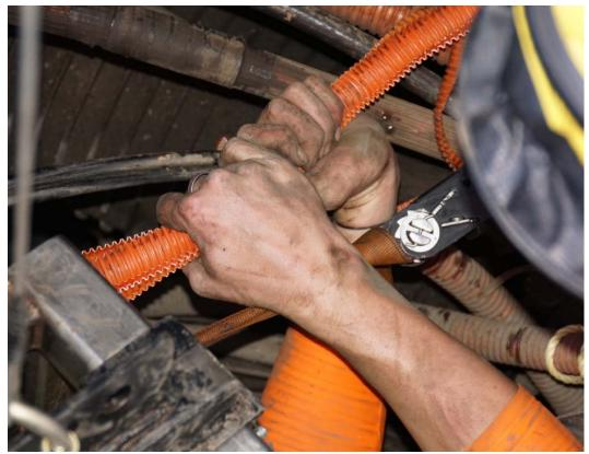
MaxSpace Recovery process: The first innerduct is being split and pulled out of the ductbank.
