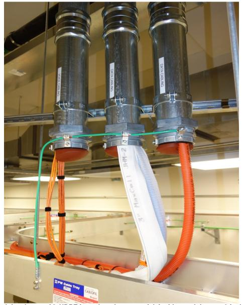
Conduits shown with HDPE innerduct that may stick inside conduit up to 6-inches.
