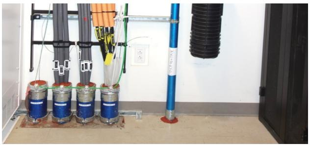
Cables routed down a wall to floor conduits shall be mounted to vertical Ladder Rack for support.
