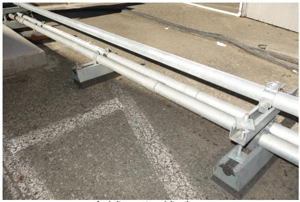
Asphalt support conduit pathway.
