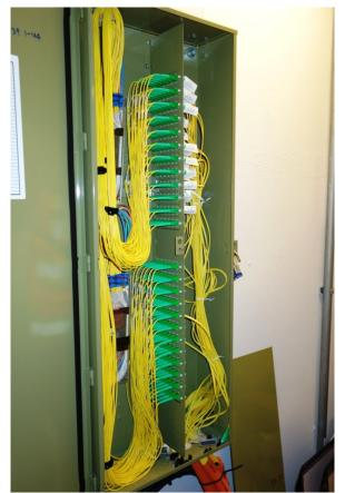
Side view of a wall-mount fiber panel showing each pigtail labeled with fiber strand number.
