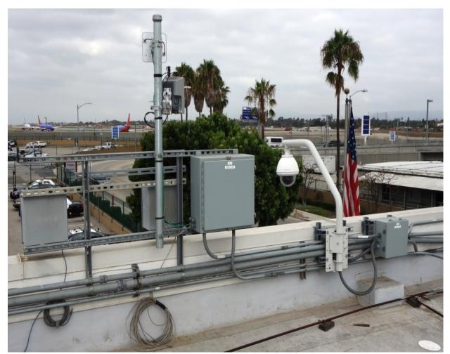
Parapet wall antenna and conduit pathway.
