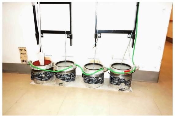
Metal conduit bushings shown with grounding wires.
