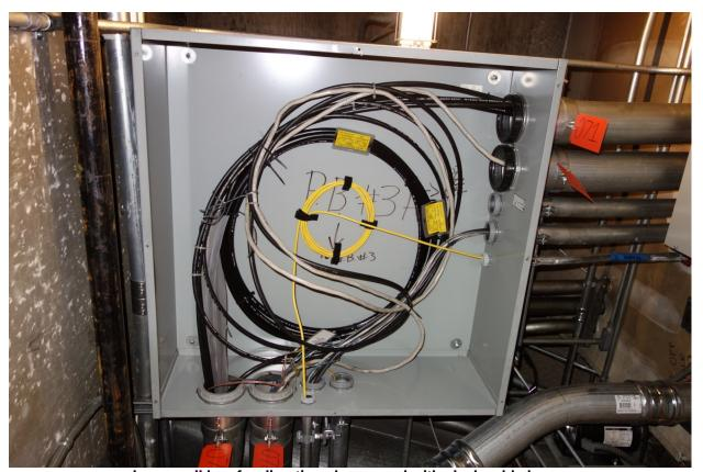
Large pull box for direction change and with slack cable loops.
