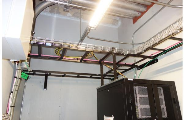
Wire Basket for fiber jumpers is shown attached to Ladder Rack. Cable waterfalls are required.
