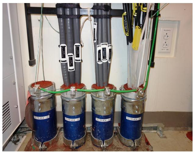
Conduit stub-ups shown secured to floor-mounted strut.
