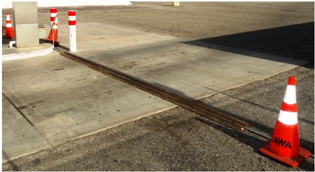
Conduit-protector at fuel pump protecting conduit.
