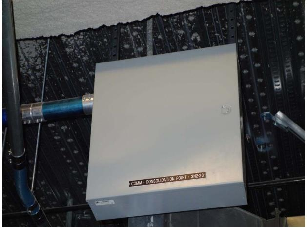
Consolidations Points may be installed in separate junction boxes in the ceiling.
