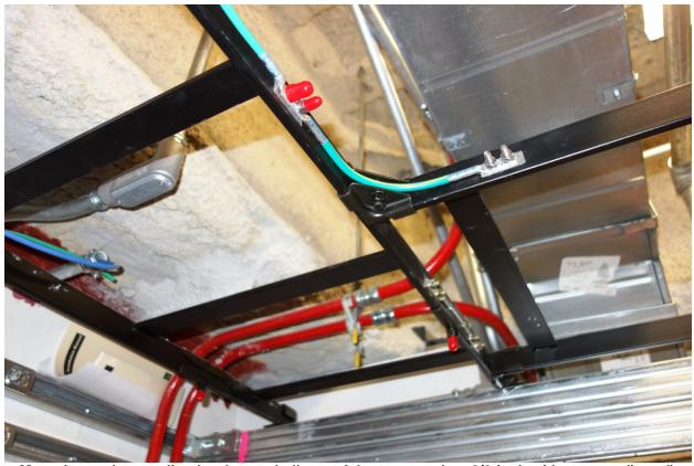
Mounting and grounding hardware shall not stick out more than 3/8-inch without caps (in red).
