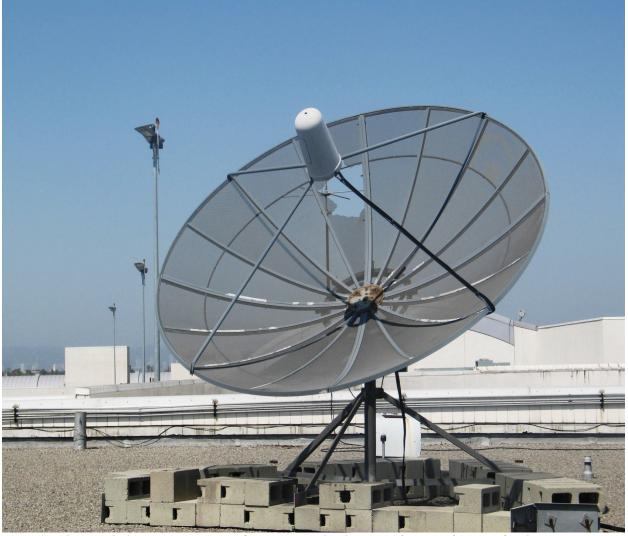
A sample large non-penetrating rectangular-base surface roof mount is shown.
