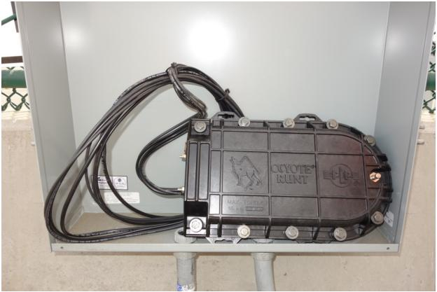
An intermediate outdoor splice case on a long fiber run shown in a junction box.
