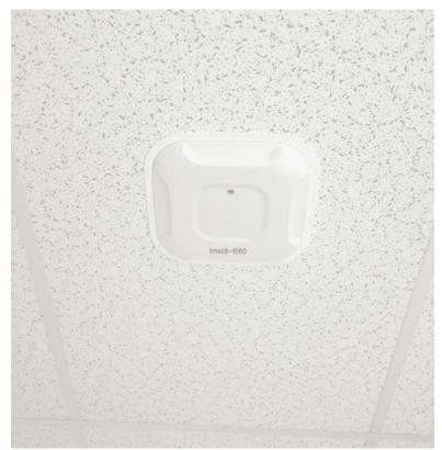
A/P mounted within ceiling tile on the suspended ceiling T-Bar.
