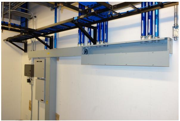
Wireway can be used for aggregate cabling of an IT system. Pull strings are required for conduits.
