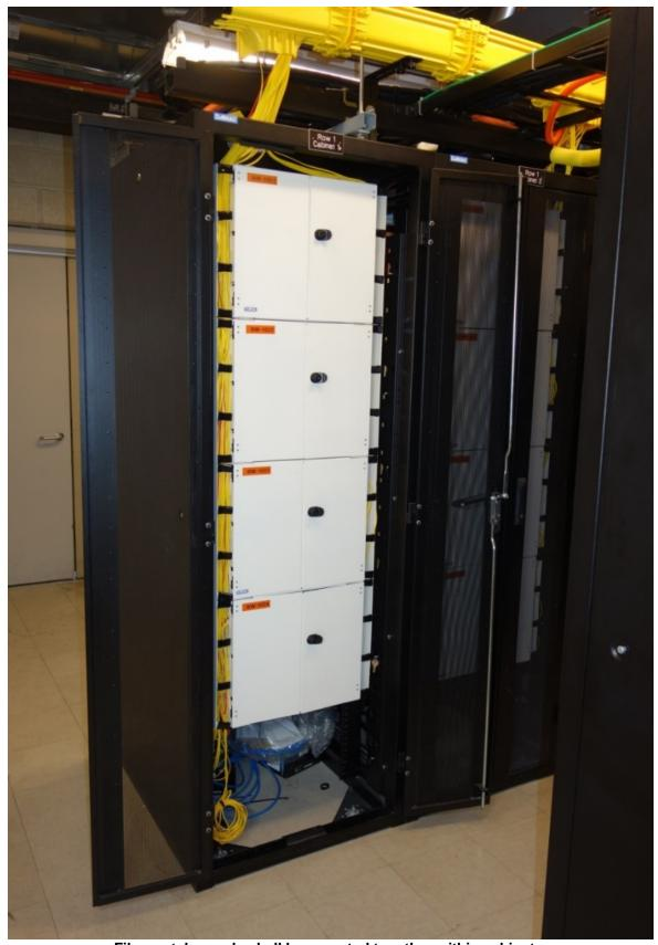
Fiber patch panels shall be mounted together within cabinets.
