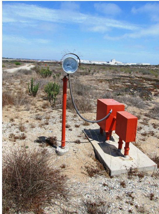
2. View of flashing Station facing east.
