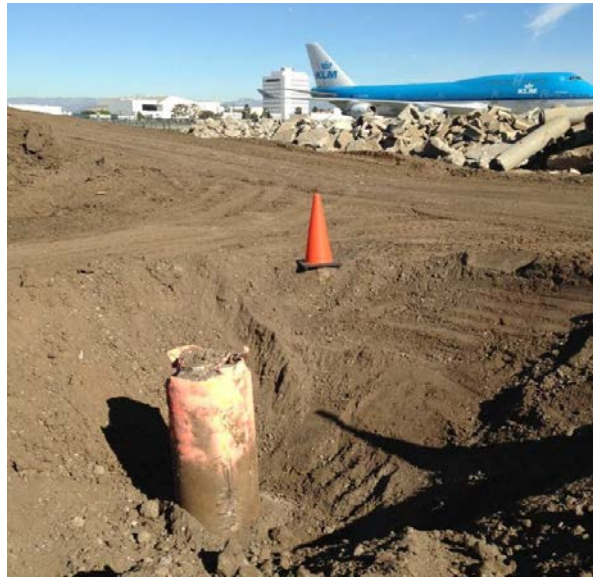
Abandoned Oil Well at LAWA WAMA construction site
