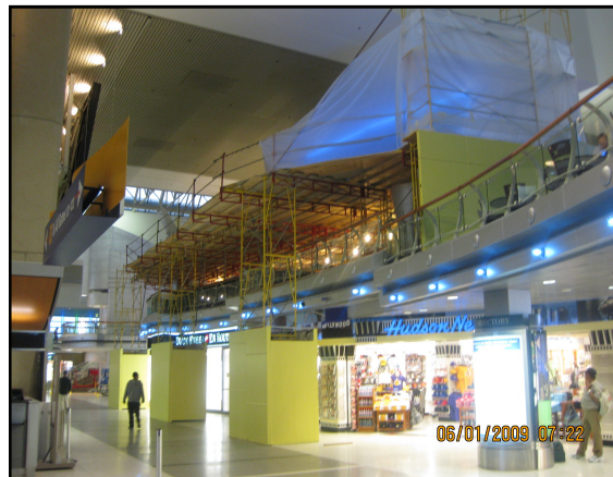
Renovation of the mezzanine bar.
