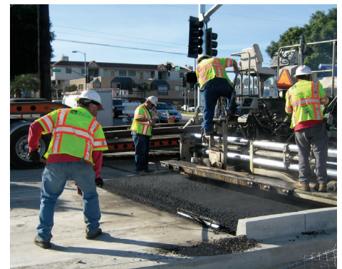
Workers resurface traffic lanes along Imperial Highway. Roadwork will improve traffic flow and alleviate congestion associated with LAX construction projects.
