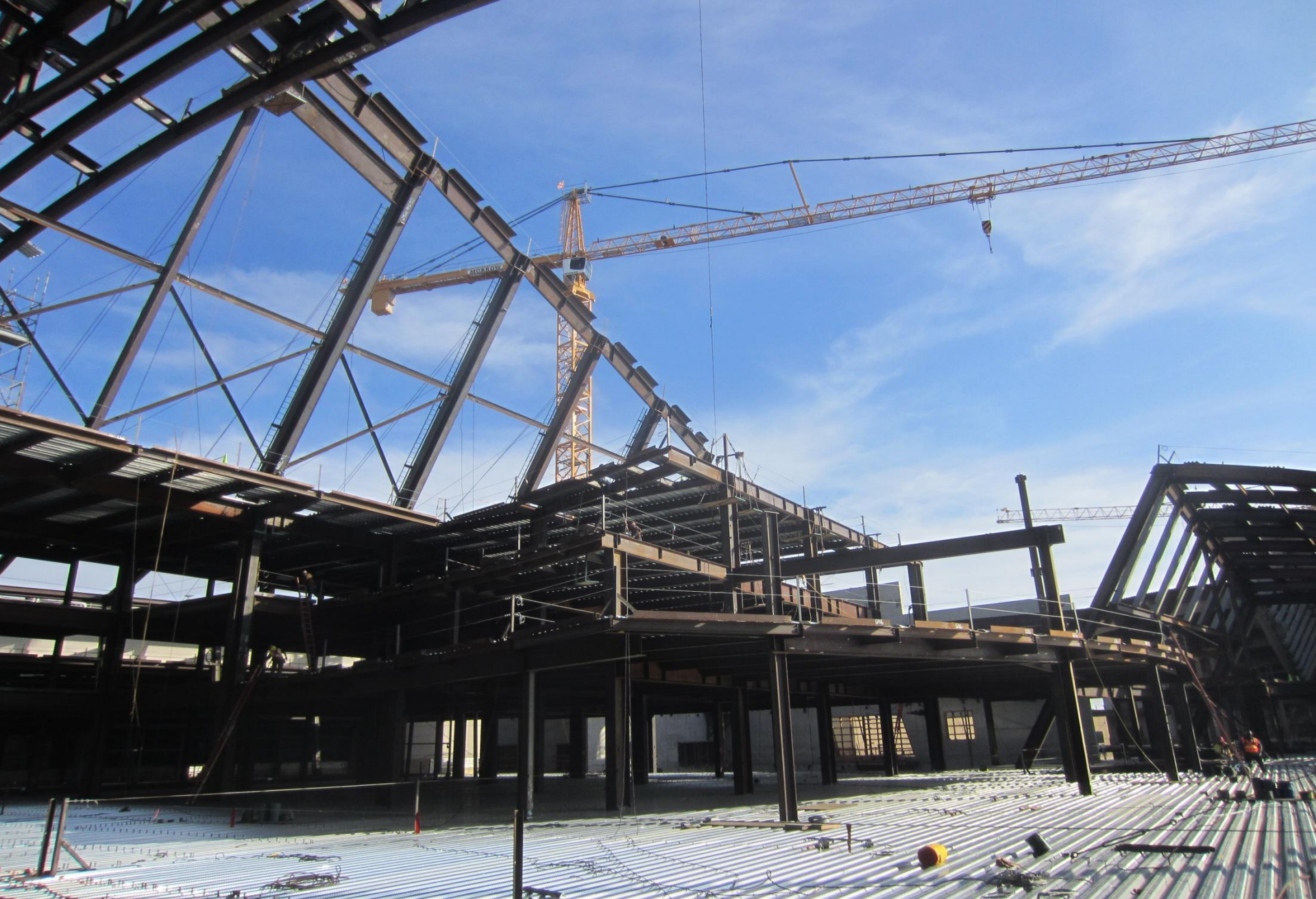
Erection of steel for the third and final bay of the core nearing completion. January 20, 2012
