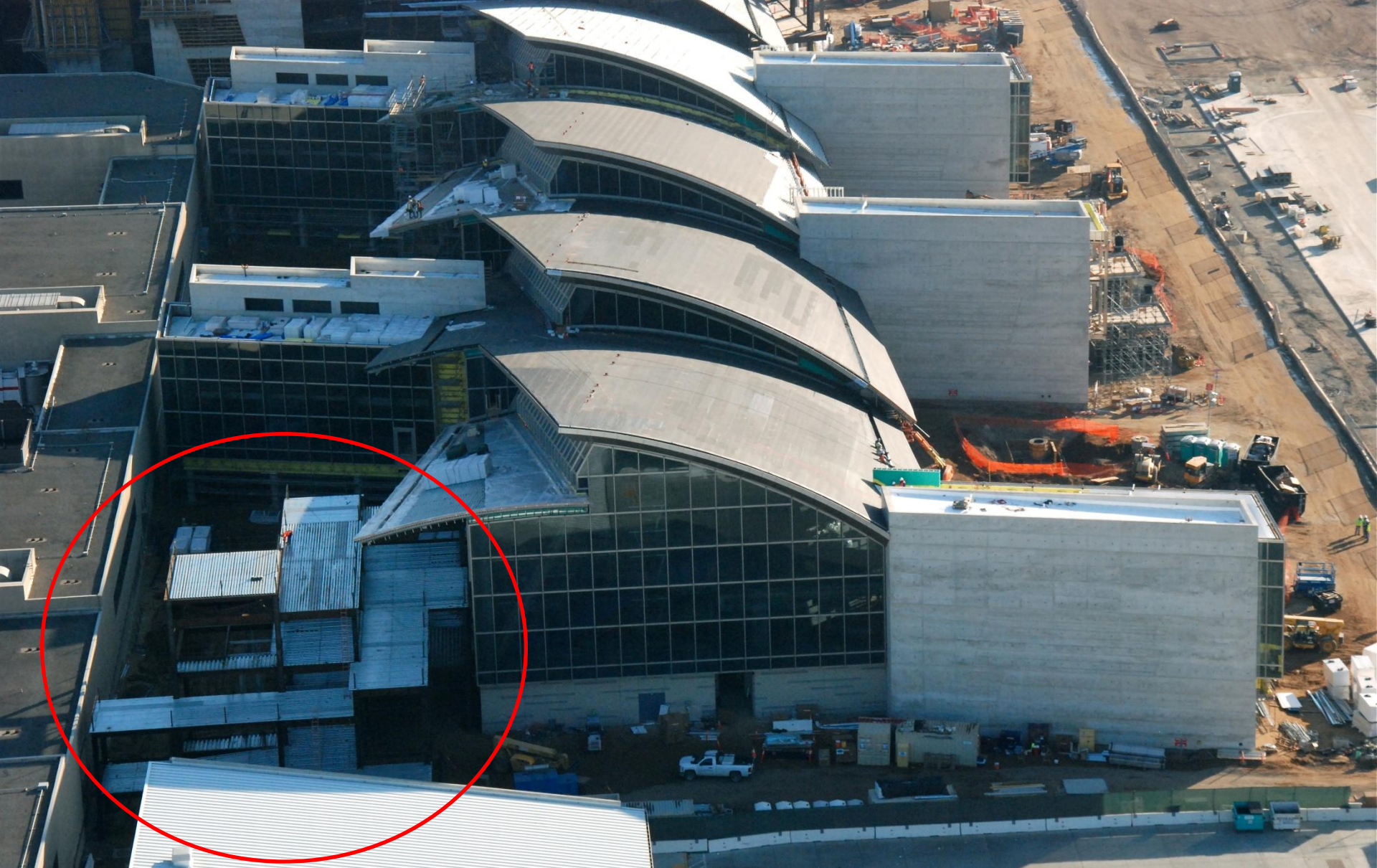
Another view of the temporary connector between the old and new concourses. This aerial also highlights how much glass the building will have and the wave-like appearance of the roofline.
