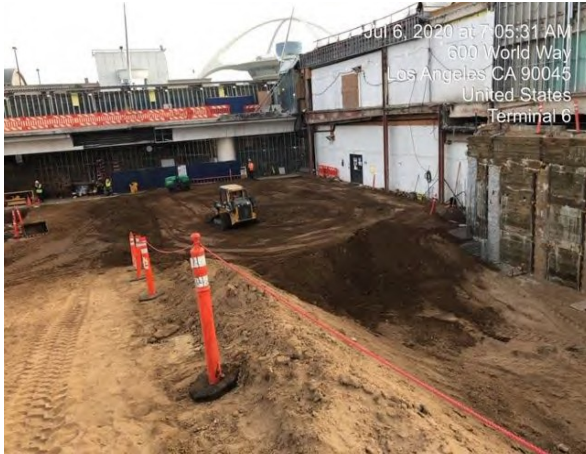
Building pad in preparation for foundation excavation
