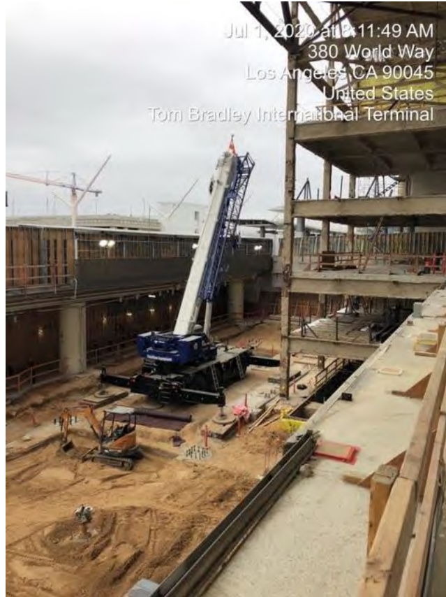
Crane in place - Formwork and rebar for grad beam concrete placement
