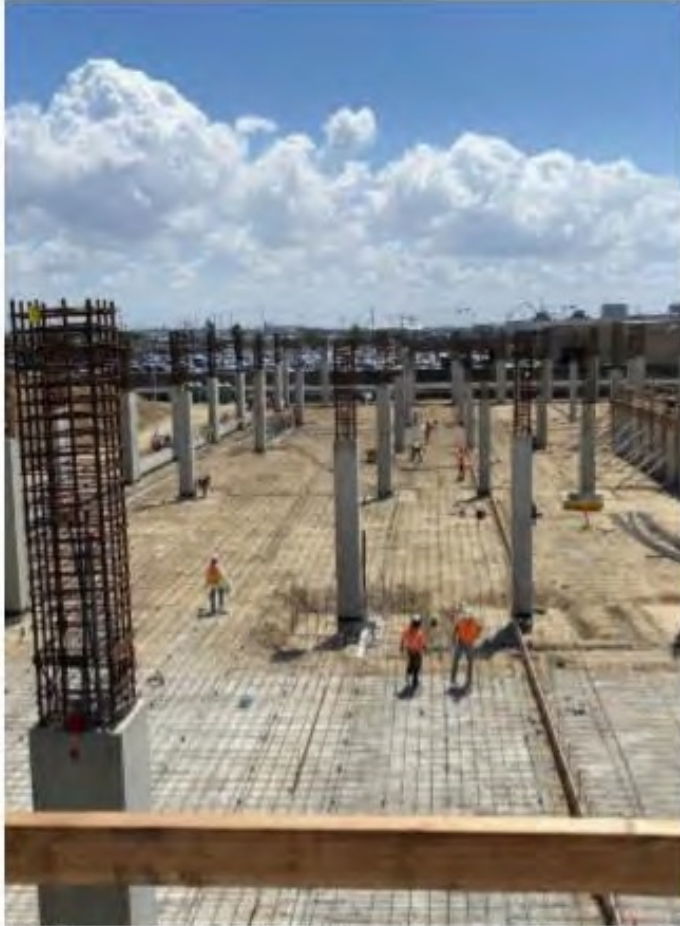
Building E – Looking East – Rebar ready for concrete placement
