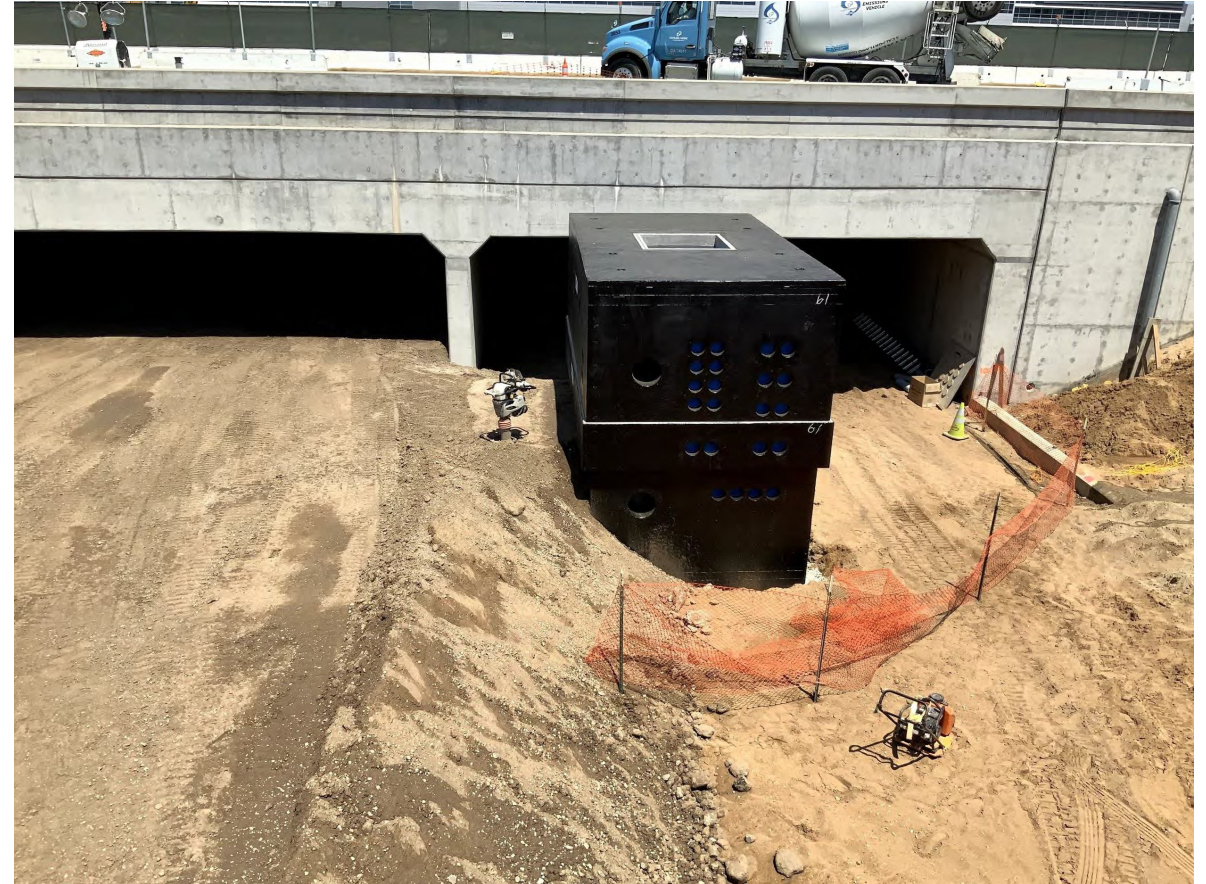
Conduit Installation and backfill on World Way West
