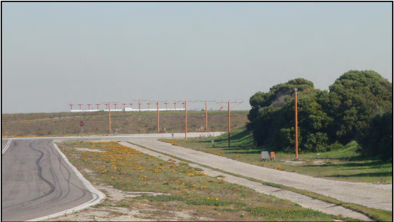
a. Existing Approach Light System (Towers) at South Airfield Runway 7L (Looking West).
