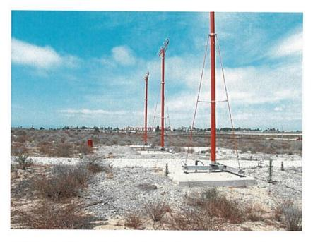
1000 foot light bar with steady burning lights to be relocated to the east of Pershing Drive. Concrete pads to remain in place.
