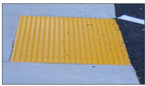
Standard plan- S-442-4 truncated dome pattern per BOE standard plans for curb ramps
