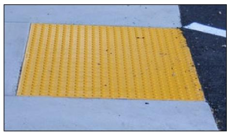
Standard plan- S-442-4 truncated dome pattern per BOE standard plans for curb ramps
