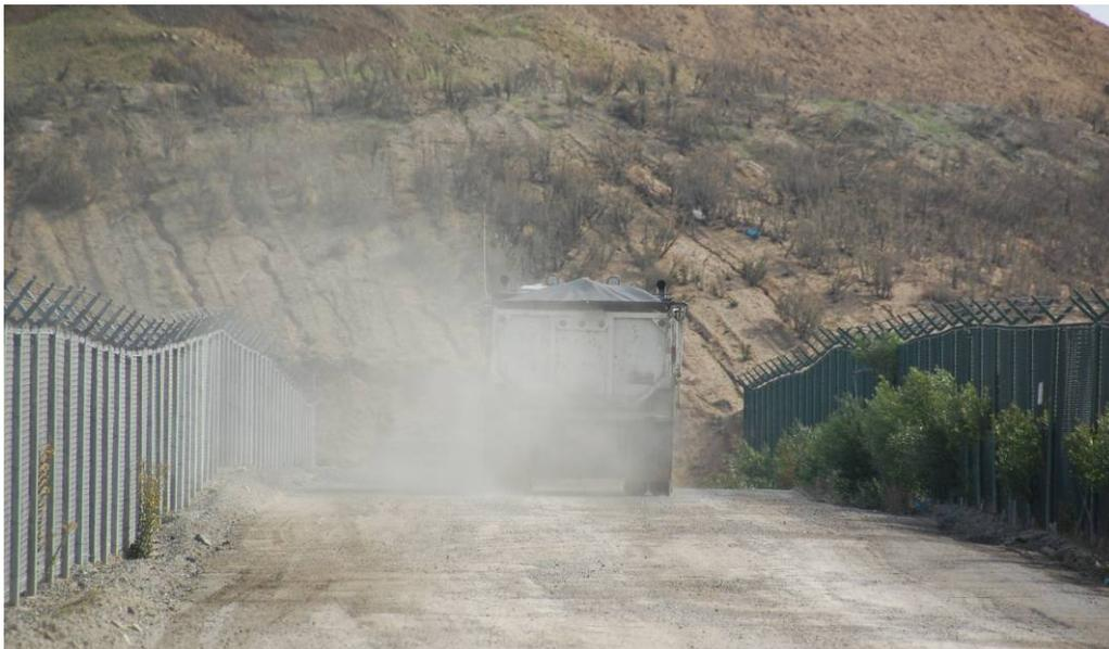
*Figure 6.-6 Excessive Dust Emissions Created During Hauling Operations*
