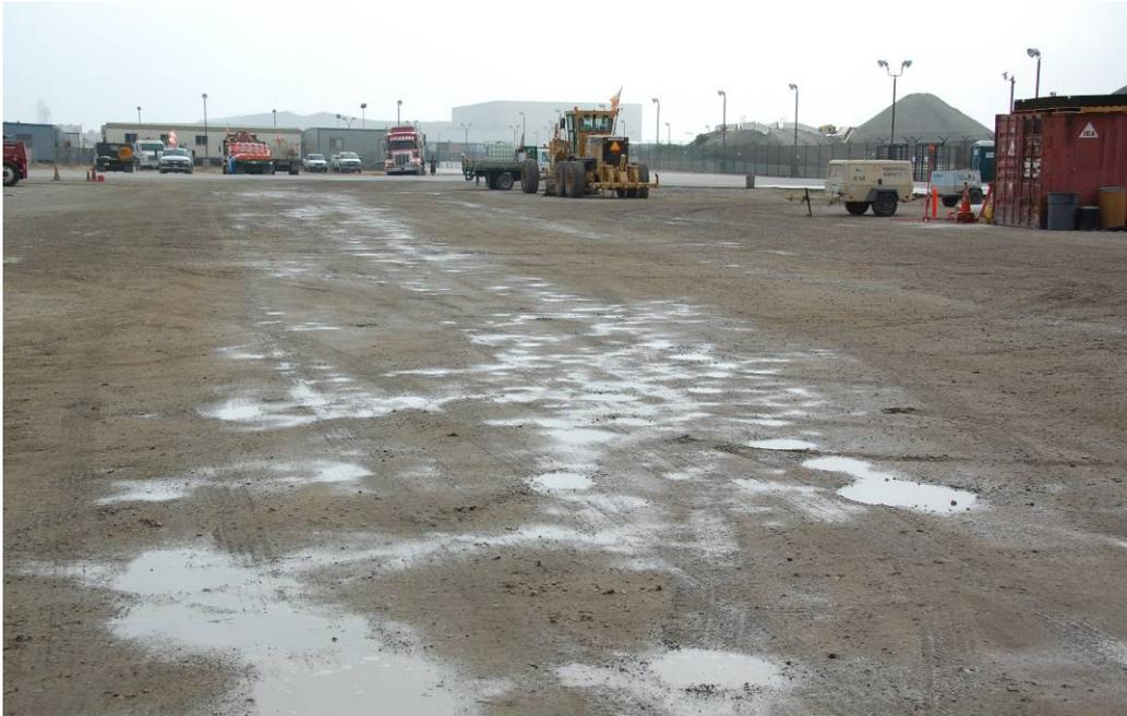
*Figure 6-5: Construction Areas are Kept Wet to Reduce Fugitive Dust Emissions*
