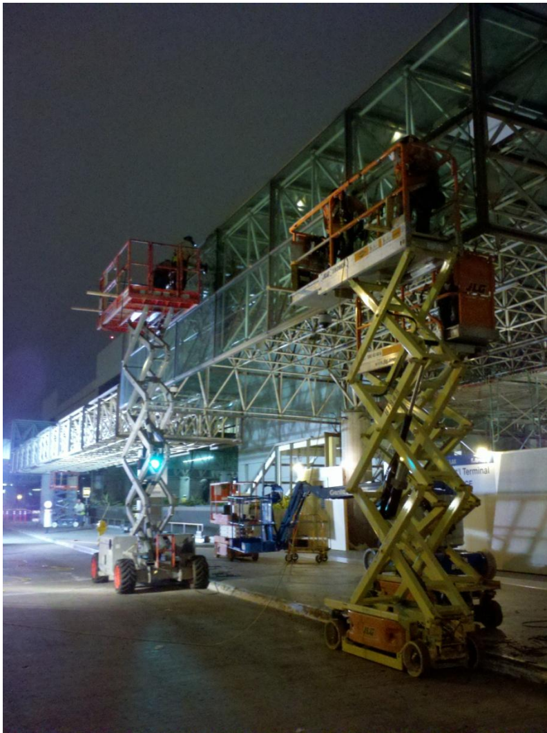
Workers removing the existing glass canopy at the “Front Door” of TBIT (upper level). August 2, 2012
