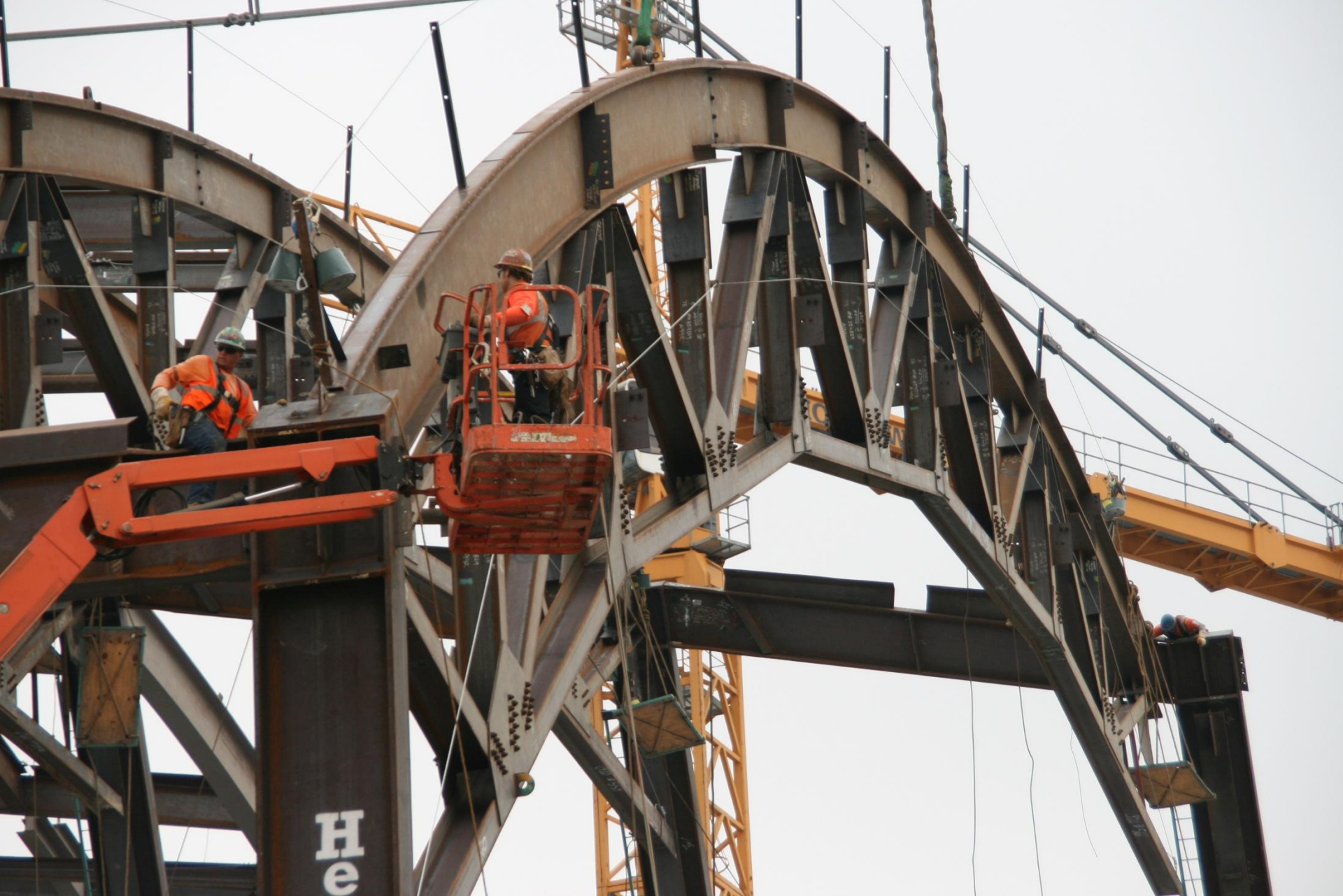
Ironworkers guiding the truss into place. August 12, 2011
