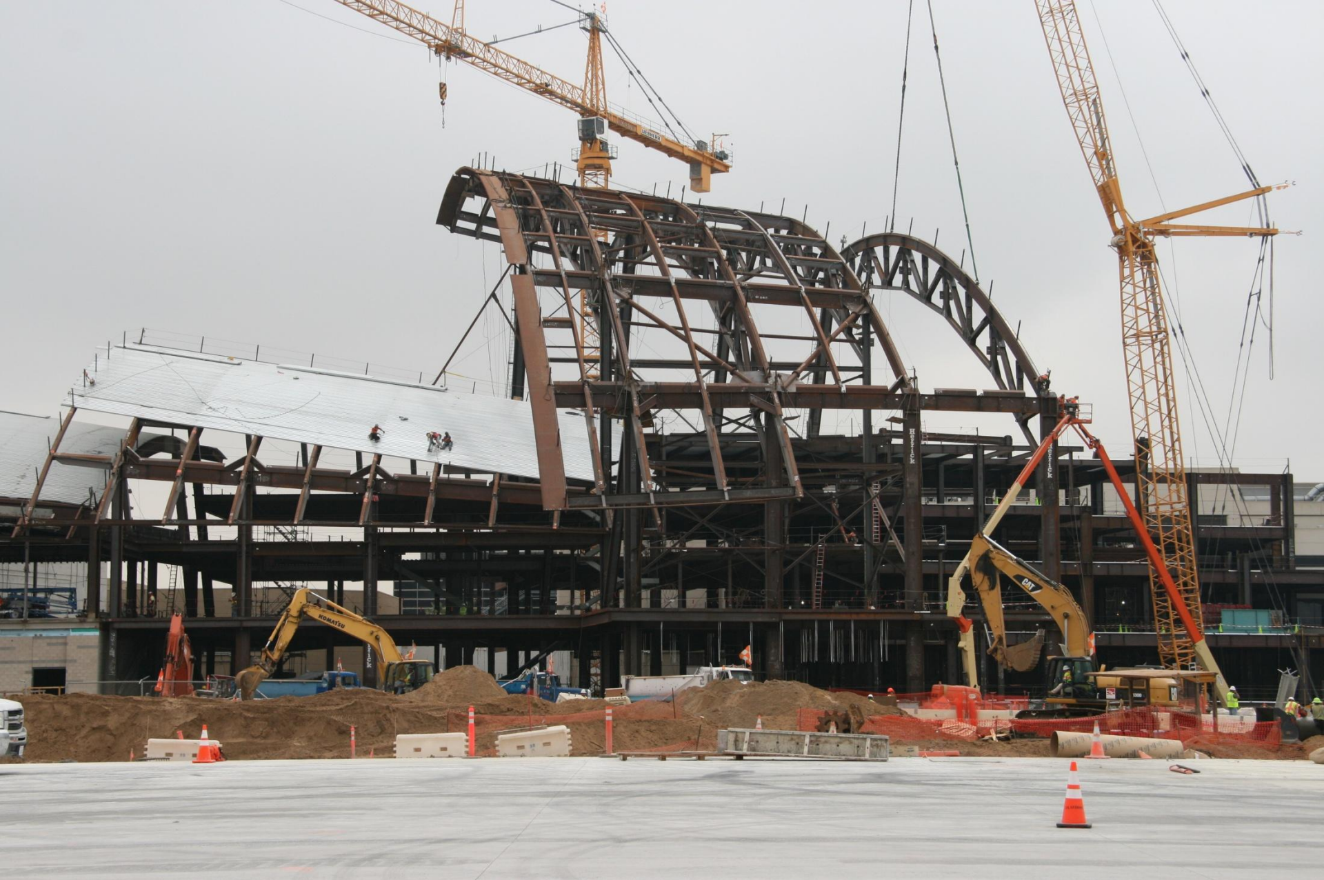
Large truss being set in place in the northern bay of the core. There will be three bays in the core each containing seven trusses.
