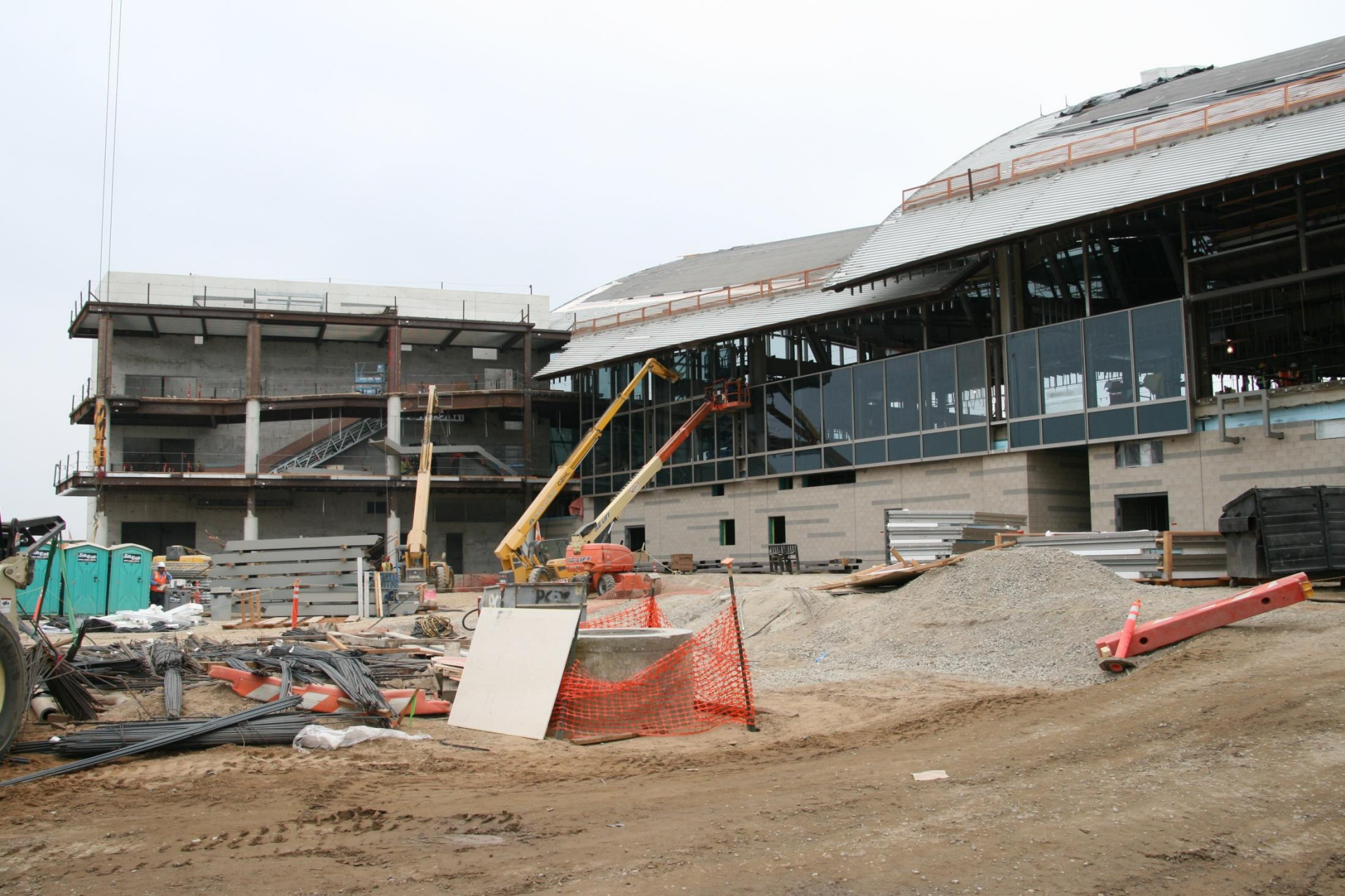
Glass curtain wall being hung in place on north concourse. August 12, 2011
