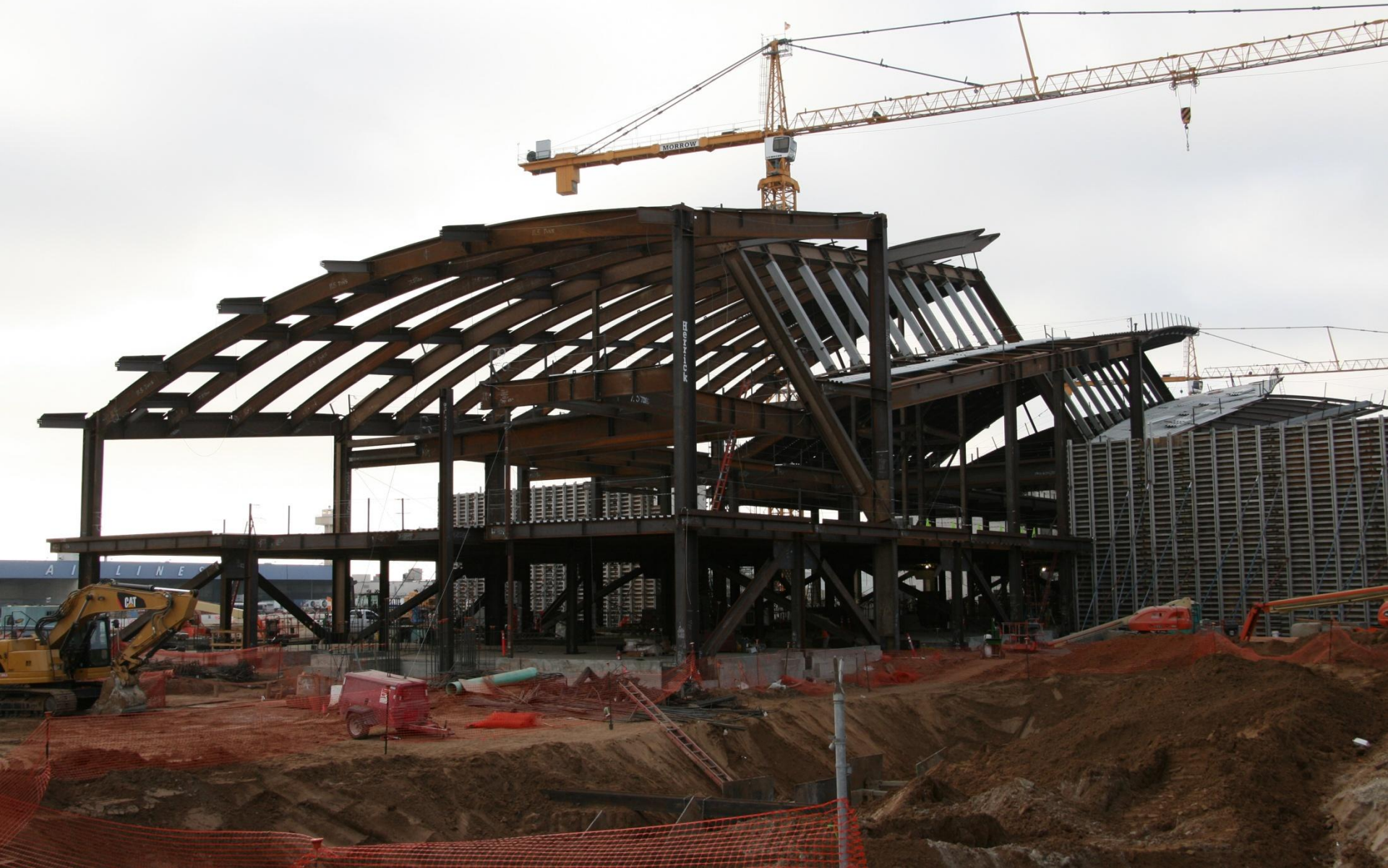
Steel for the final bay of the south concourse is now set. August 9, 2011
