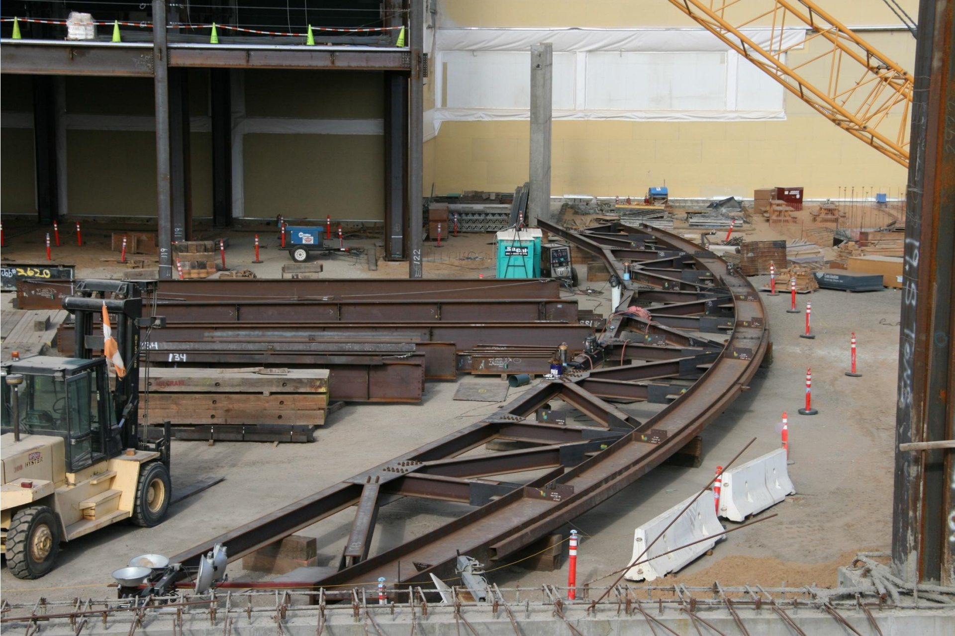
Core roof truss in laydown area prior to being hoisted into place. August 9, 2011
