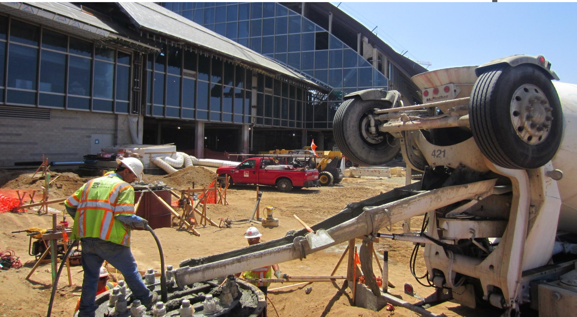
Concrete being poured into the support structure for the jet bridges at Gate 130. May 17, 2012
