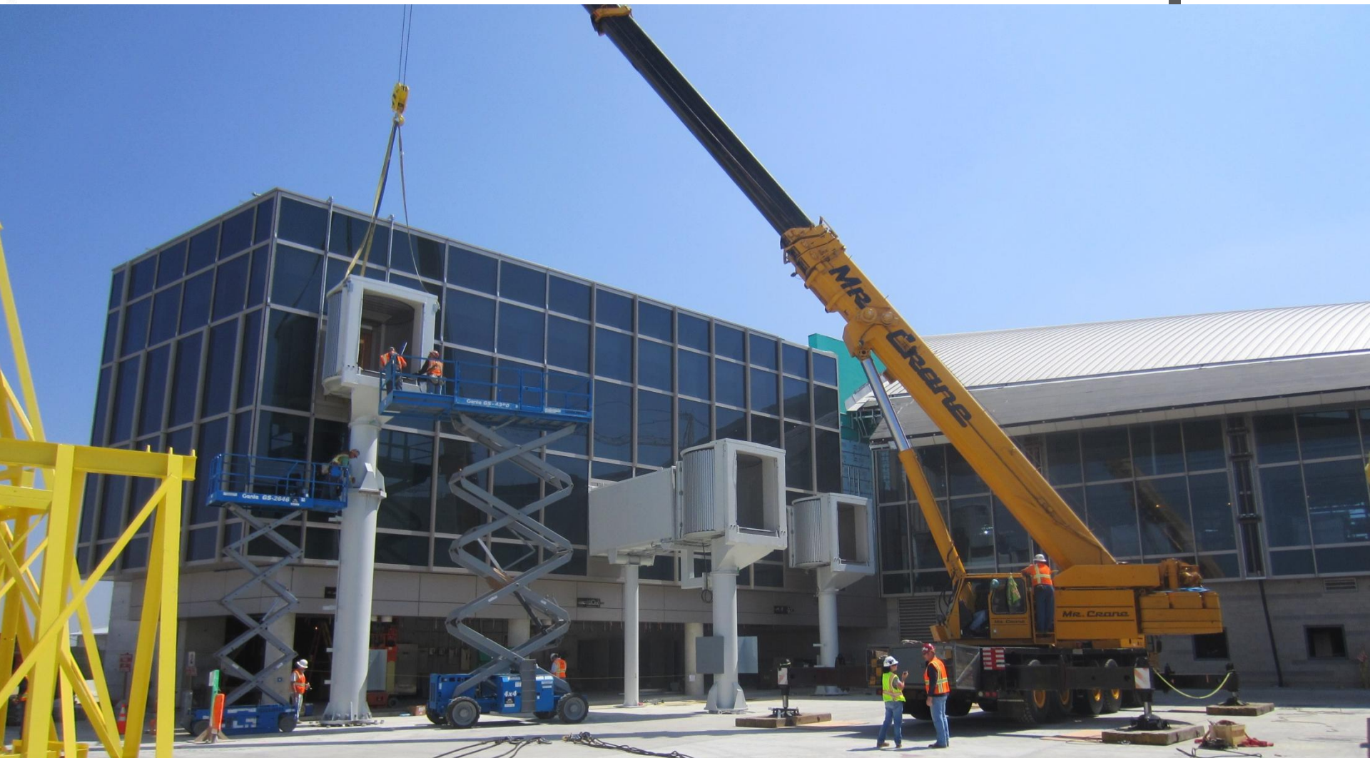
Jet bridge access points being installed at Gate 134. May 17, 2012
