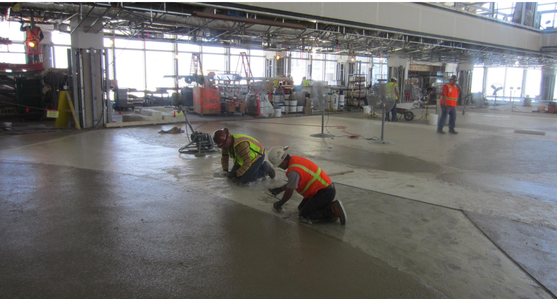
Workers surfacing the terrazzo flooring. May 17, 2012
