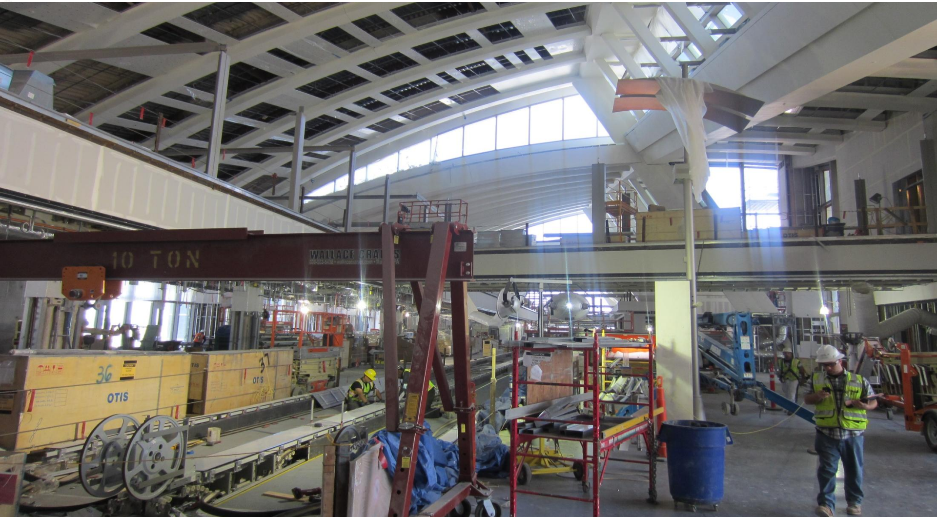
Interior of the north concourse. Moving walkway and ceiling panels being installed. May 17, 2012
