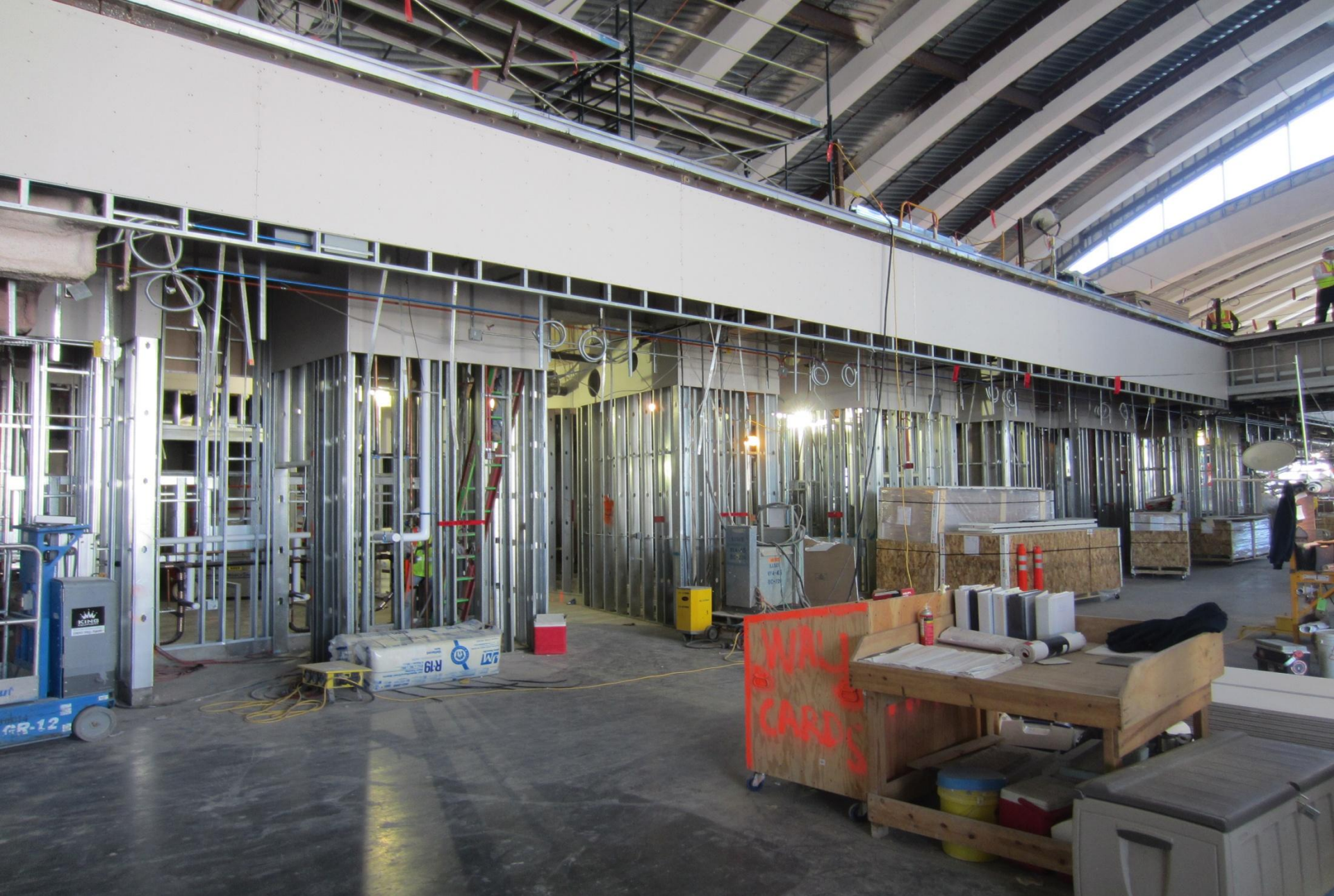
The aluminum framing for the walls of the restrooms in the north concourse. March 8, 2012
