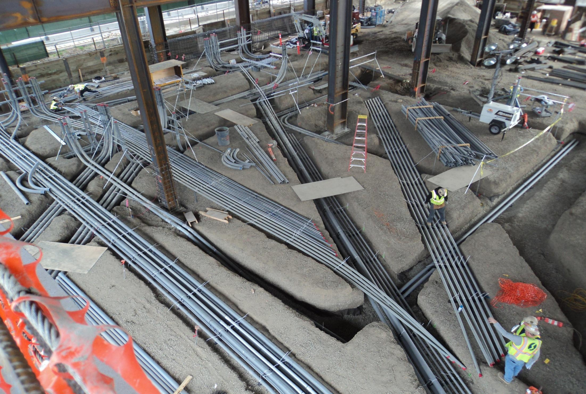
“Serious” conduit being installed in the new Central Utility Plant (CUP). February 21, 2012
