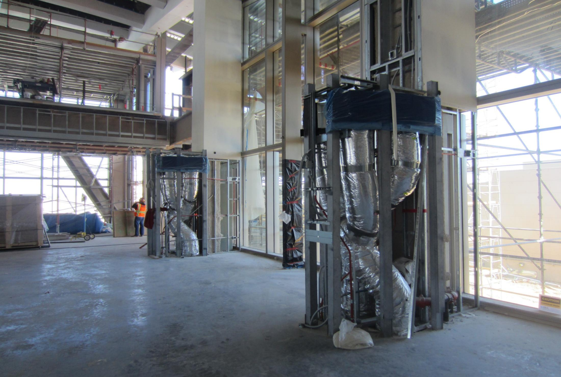
Installation of the ventilation system for the north concourse. March 8, 2012
