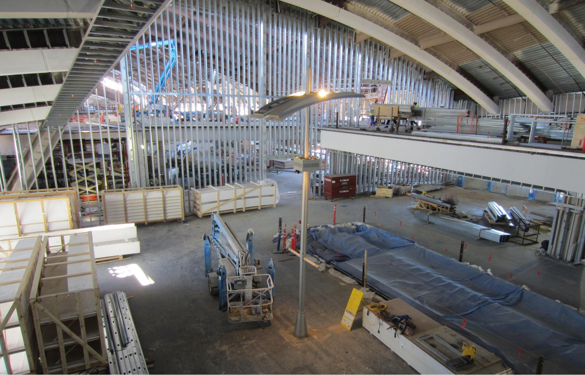
Aluminum framing for the temporary wall separating the Great Hall and the north concourse. This temporary wall will allow the north concourse to open while the Great Hall is still under construction.
