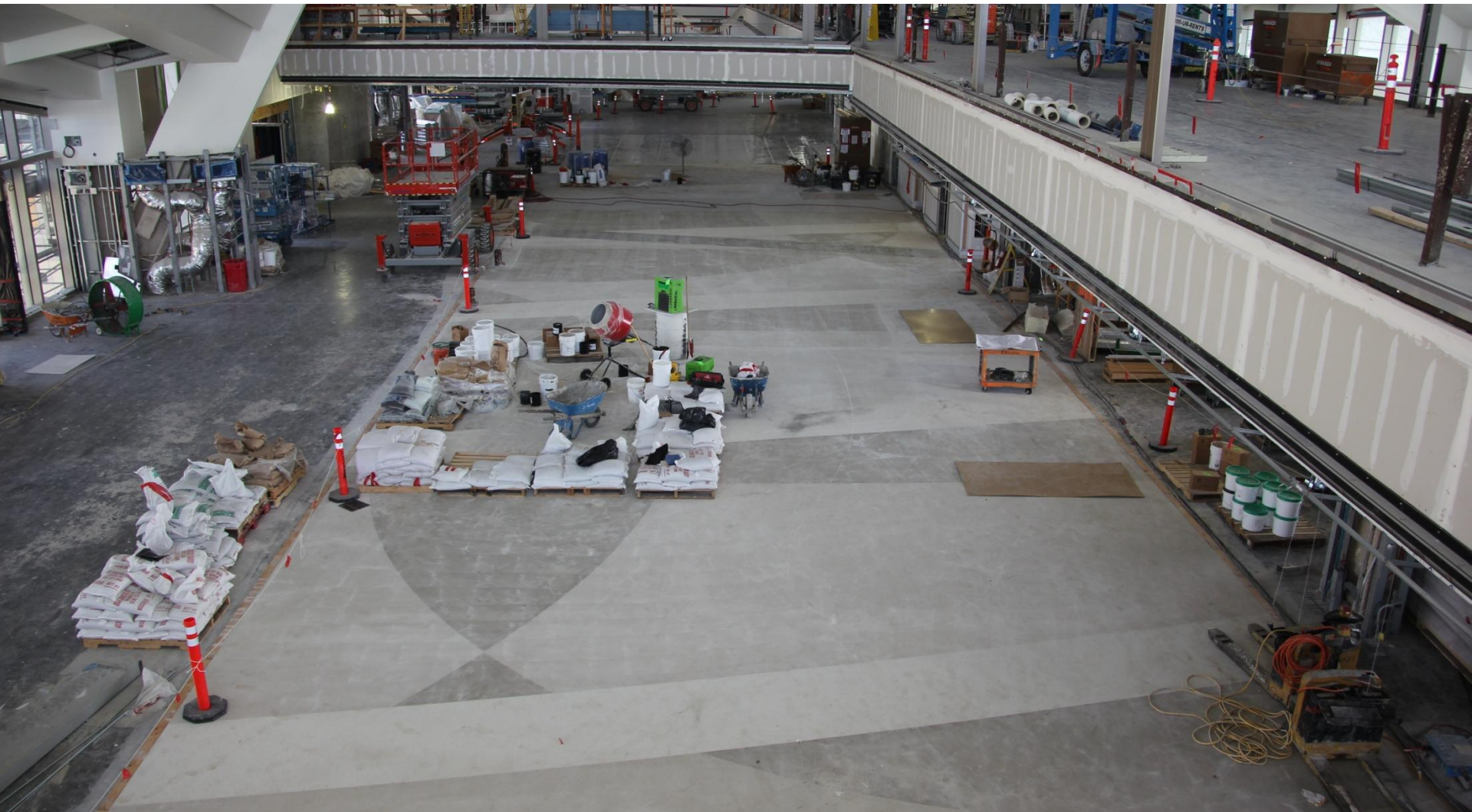
The terrazzo flooring is being installed on the departure level of the north terminal. June 1, 2012
