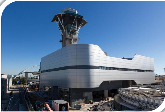
This project provides a replacement Central Utility Plant (CUP) to the one that has been in operation since 1961. The new CUP will supply hot and chilled water to all terminal buildings and other facilities in the Central Terminal Area at LAX. Major project components include:
