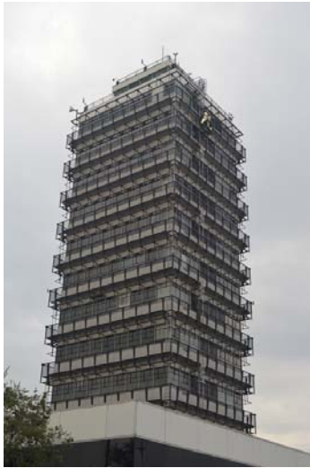
1961 Airport Traffic Control Tower
