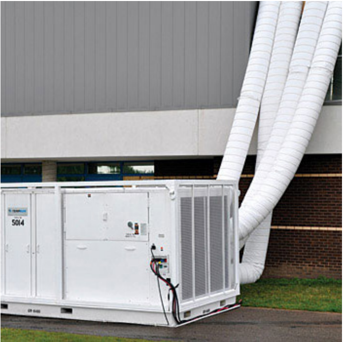
Temporary HVAC system Source: www.esmagazine.com
