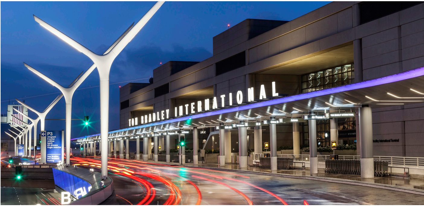
CTA Roadway Light Poles Source: www.archlighting.com/
