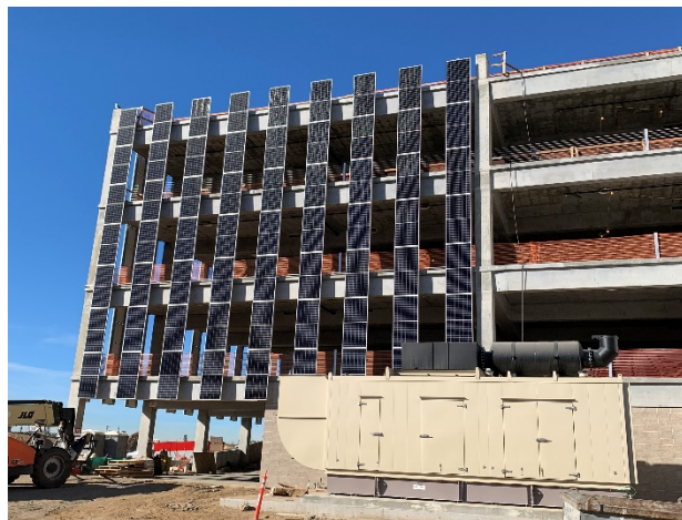
Vertical solar panels on the ConRAC Facility Idle Storage Building
