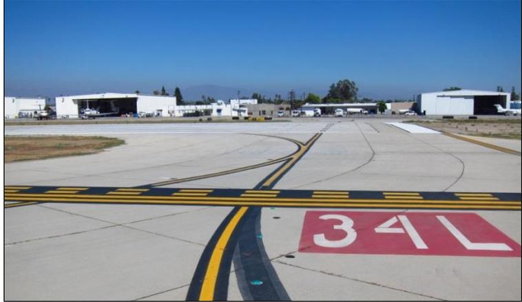
**lines** and denote a runway holding position. These markings are always co-located with a Mandatory Instruction Sign (mandatory sign). When approaching this marking from the solid side, an operator may NOT cross without first obtaining clearance from the air traffic control tower. When approaching this marking from the broken side of the line, the aircraft/vehicle MUST cross the solid lines to be clear of the runway.
