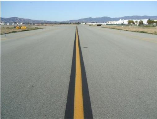
**Taxiway Centerline**—a solid yellow line used to denote the center of the taxiway and provide alignment and guidance for aircraft.
