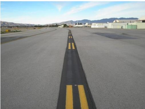
**Dashed Taxiway Edge Line**—a dashed double yellow line indicating operators **may** cross the line as there is full strength pavement on both sides of the line. Usually found where a taxiway is directly adjacent to ramp/apron area.
