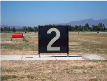
**Runway Distance Remaining Signs** have a black background with white inscriptions. Runway Distance Remaining Signs provide distance remaining information to pilots during takeoff and landing operations. The number on the sign provides the remaining runway length in 1,000-foot increments.
