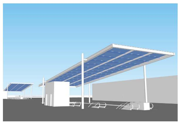
Canopy with spider glass connections with minimal structural beams
