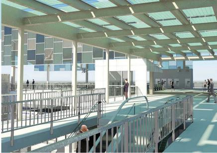
Breezeway canopy with ETFE panels (Ethylene tetrafluoroethylene)
