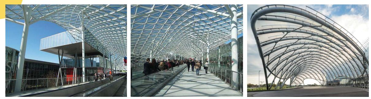
Tensile steel canopy with ETFE (Ethylene tetrafluoroethylene)
