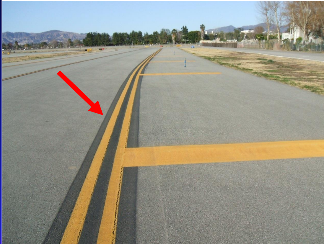
Taxiway Edge-line with Shoulder Markings
