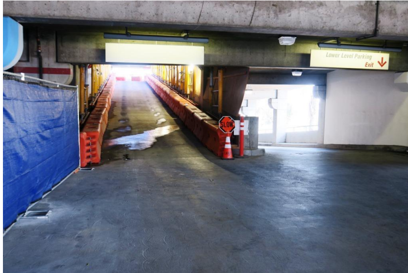
The ramp between Levels 3 and 4 in Parking Structure 4 is open, except during overnight work.
