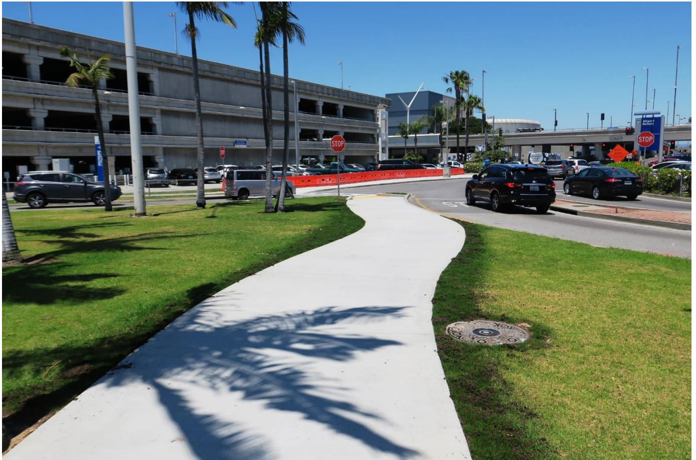
Central Terminal Area Portion of new Pedestrian Walkway between Terminals 1 & 7
