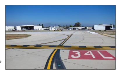
**lines** and denote a runway holding position. These markings are always co-located with a Mandatory Instruction Sign (mandatory sign). When approaching this marking from the solid side, an operator may NOT cross without first obtaining clearance from the air traffic control tower. When approaching this marking from the broken side of the line, the aircraft/vehicle MUST cross the solid lines to be clear of the runway.
