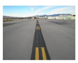
**Dashed Taxiway Edge Line**—a dashed double yellow line indicating operators <u>may</u> cross the line as there is full strength pavement on both sides of the line. Usually found where a taxiway is directly adjacent to ramp/apron area.
