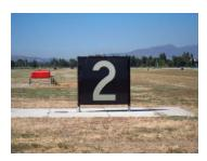
**Runway Distance Remaining Signs** have a black background with white inscriptions. Runway Distance Remaining Signs provide distance remaining information to pilots during takeoff and landing operations. The number on the sign provides the remaining runway length in 1,000-foot increments.
