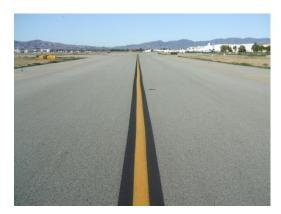
**Taxiway Centerline**—a solid yellow line used to denote the center of the taxiway and provide alignment and guidance for aircraft.
