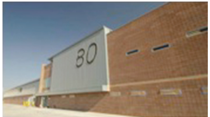
The new ARFF Station 80 has 27,500 square feet to house and maintain more personnel and equipment than the previous facility.
