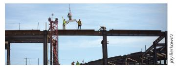
**TOPPING OUT** – Construction workers prepare to place the final structural steel beam atop the T-4 connector building's frame.
