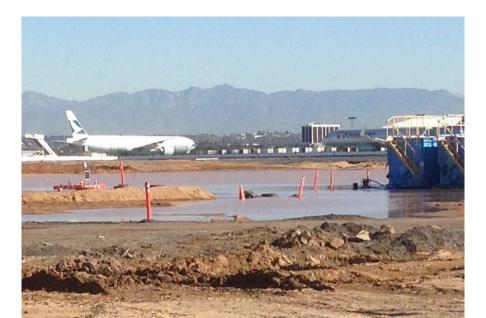
Figure 7-1: Heavy Rains Result in Standing Water on MSC Construction Site
