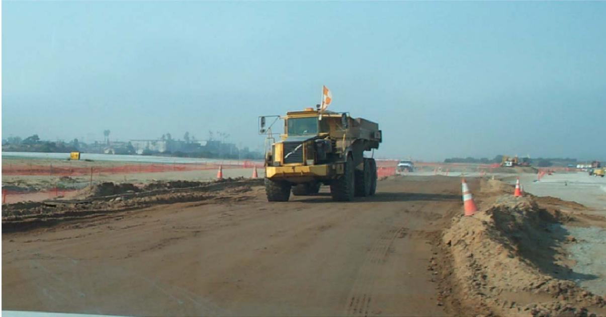
*Figure 6-14: Haul Roads are Kept Wet to Reduce Fugitive Dust Emissions*
