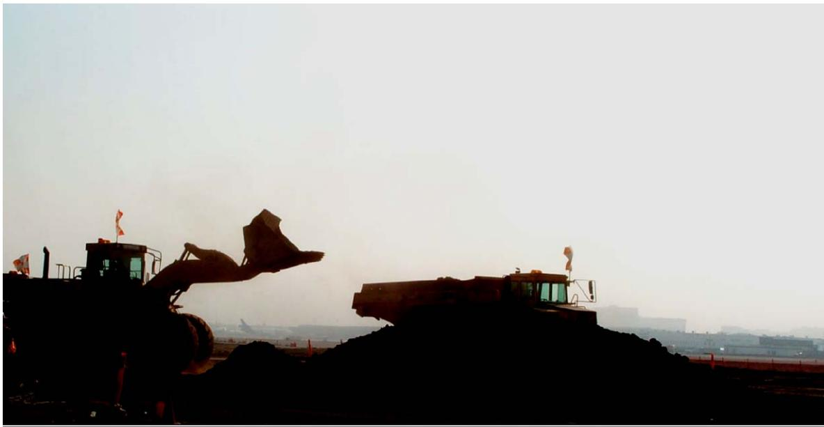
*Figure 6-17 Excessive Dust Emissions Created During Loading Operations*
