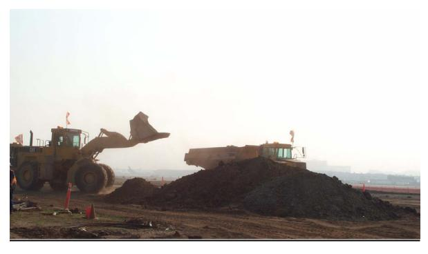
Figure 6.-8 Excessive Dust Emissions Created During Loading Operations
