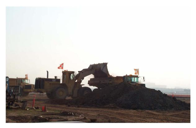
Figure 6.-7 Excessive Dust Emissions Created During Loading Operations
