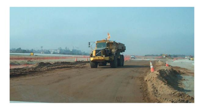
Figure 6-6: Haul Roads are Kept Wet to Reduce Fugitive Dust Emissions
