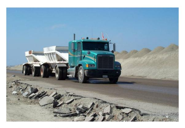
Figure 6.2-12: Haul Roads are Kept Wet to Reduce Fugitive Dust Emissions
