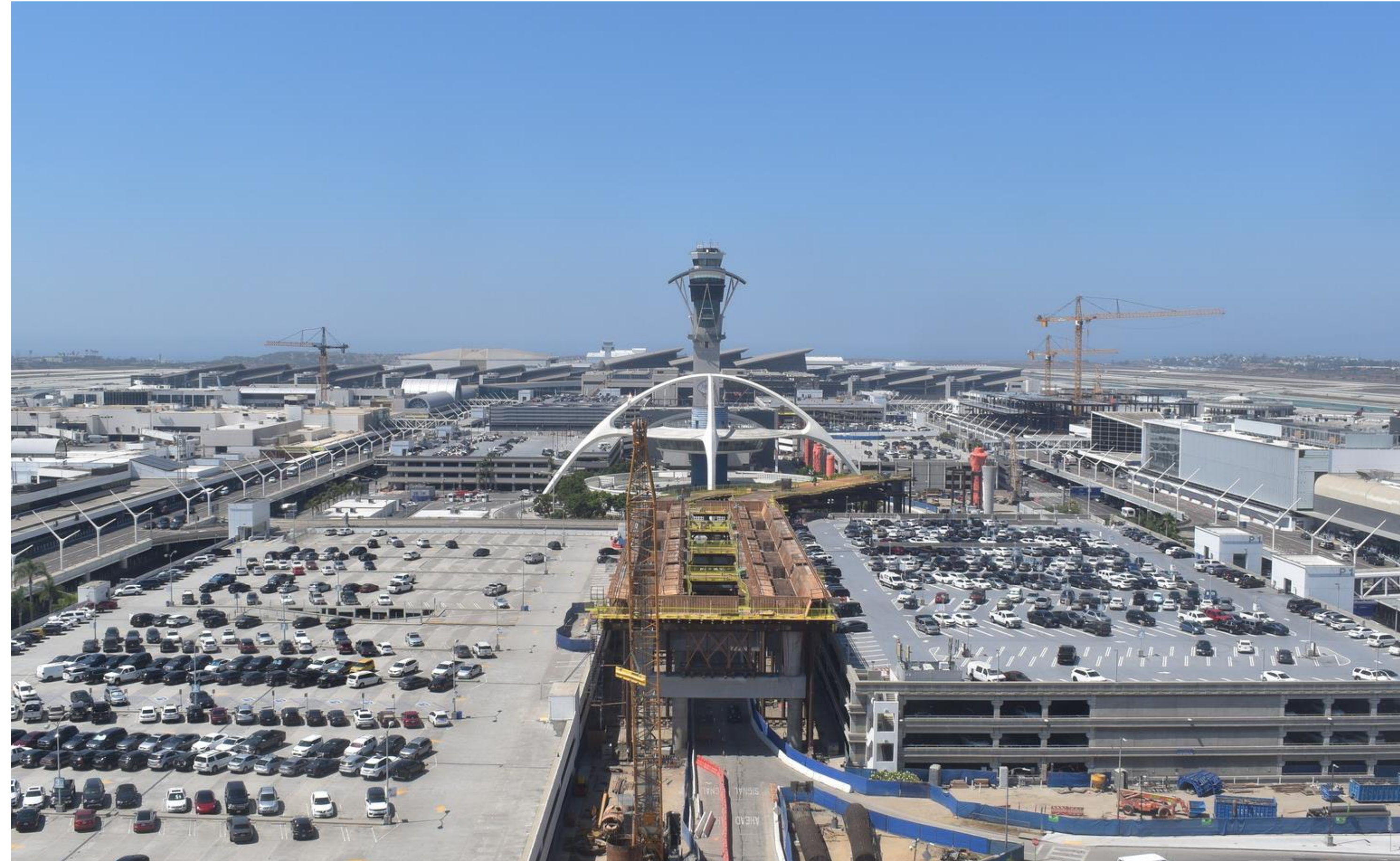
CTA East APM Station Construction
