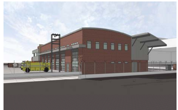
The new ARFF accommodate seven rescue and emergency response vehicles.
