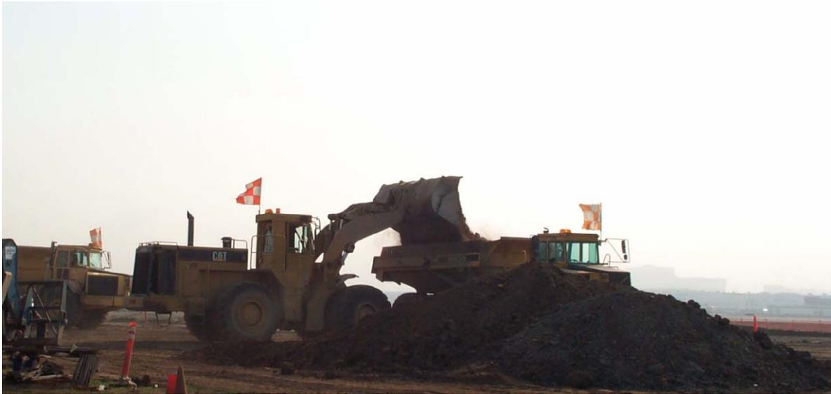
*Figure 6-16 Excessive Dust Emissions Created During Loading Operations*
